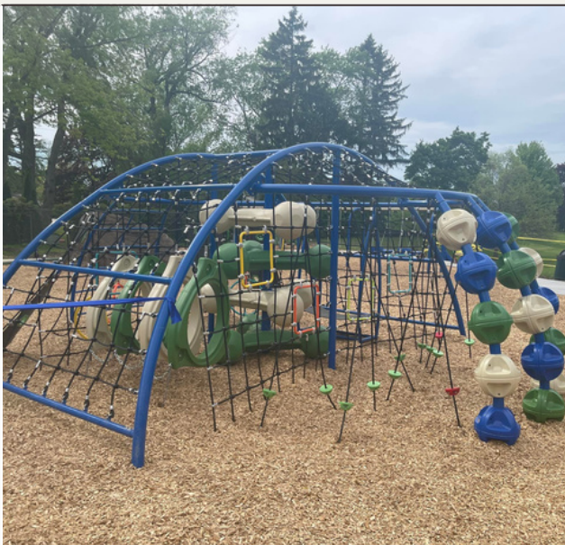
Ellsworth Park Playground Renovation
