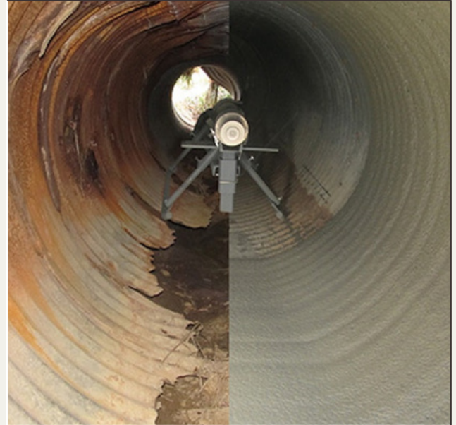
Sanitary Sewer Rehabilitation Project
