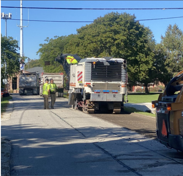
Road Resurfacing and Stormwater Project
