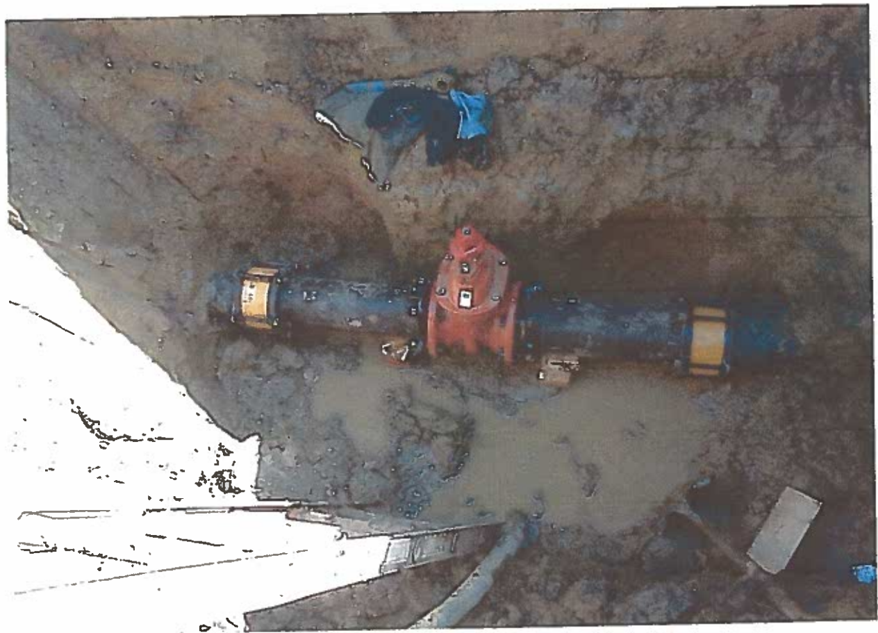
New 6" line valve and couplings
