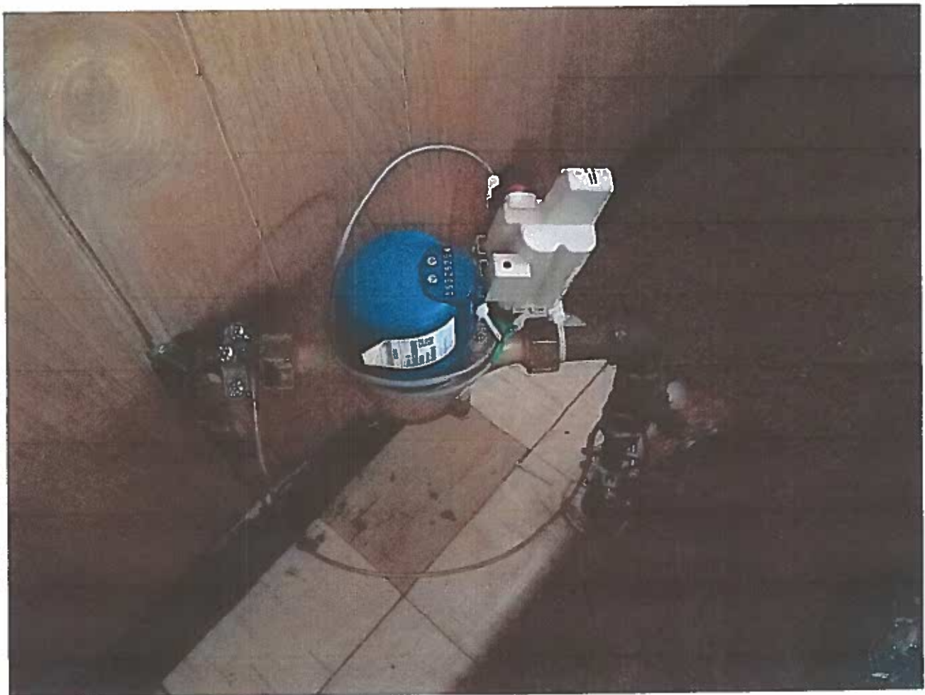
New Hersey water meter with an Itron radio
