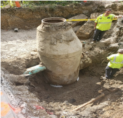
245 Logan (rerouted sewer lateral line)
