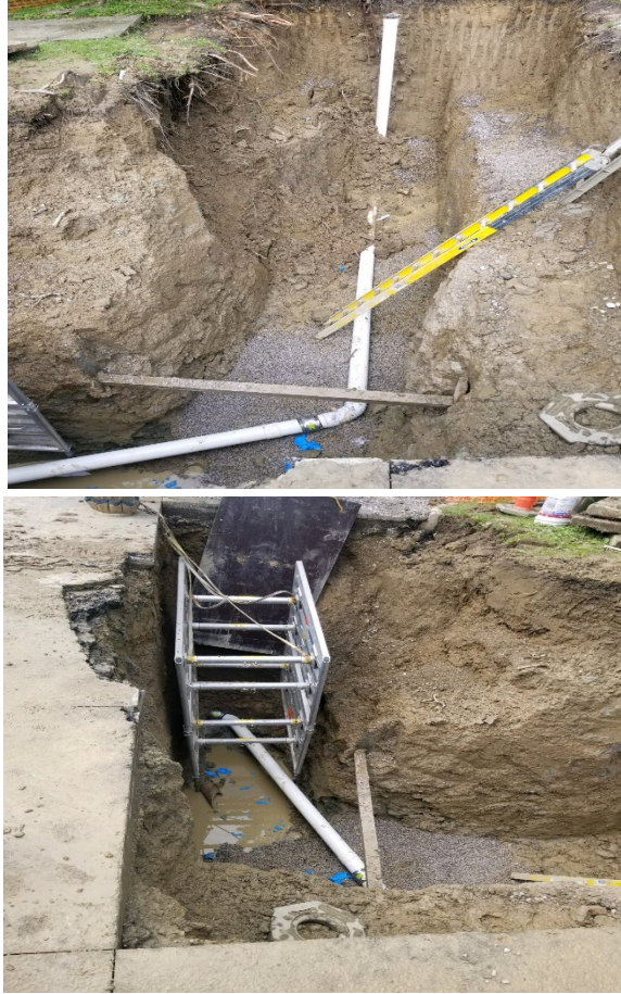
29 W. Interstate (replace from test tee to Main and Road )
