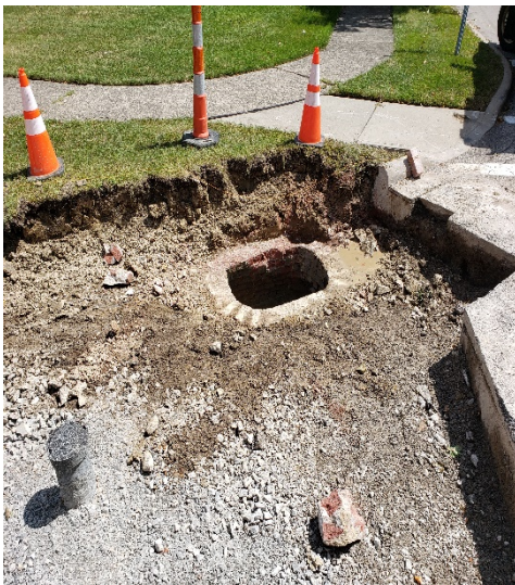
Heather at Briar ( catch basin repair )
