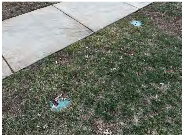
Additional irrigation control access, east side of subject property
