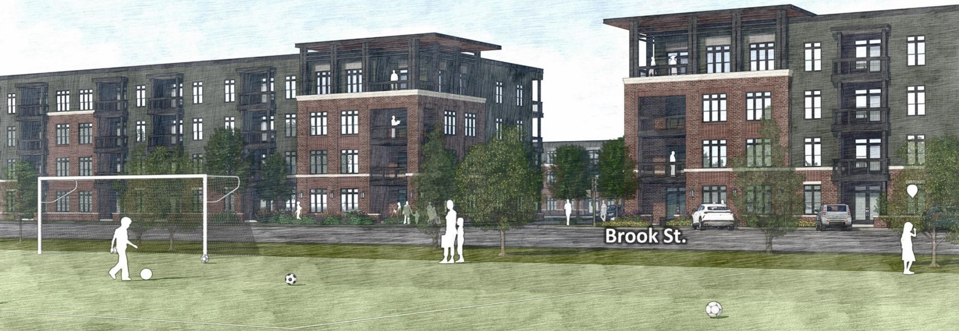
BUILDING C AND D FROM EBB GANTT PARK
