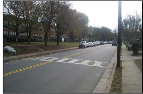
Figure 30 The existing crossing north of Harris is at a mid-block crossing, where motorists are less likely to anticipate pedestrians.
