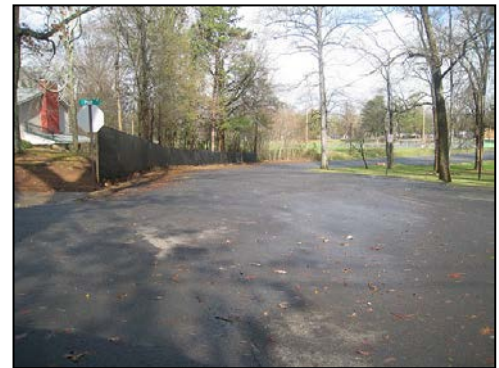
Figure 26 Park Drive is relatively wide as it goes through Davis Park, a condition that can encourage speeding.
