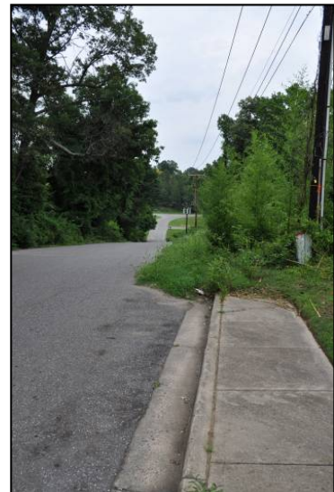
Figure 16 Sidewalk on Vine Street ends just east of Flowers Court.
