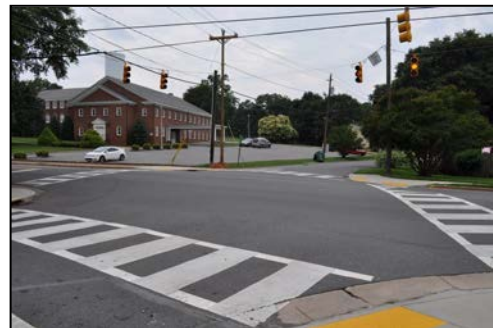
Figure 31 There are no pedestrian countdown signals at the Myrtle Street intersection and the north crossing is skewed.
