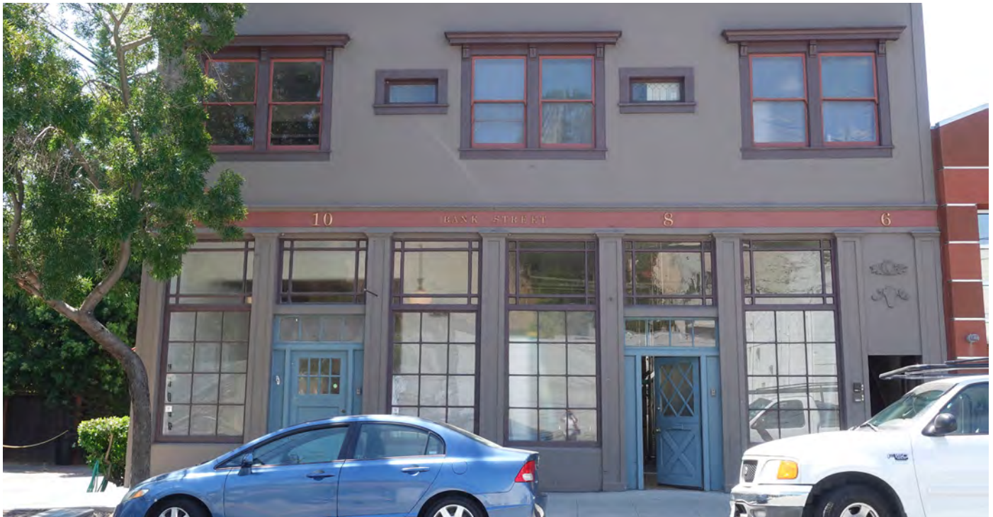
Example of a Maker Shopfront
