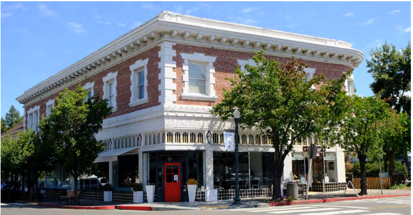
Example of Main Street Building
