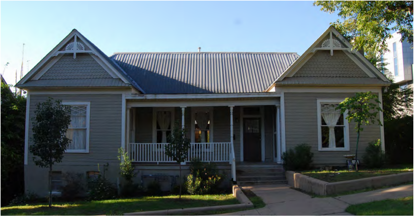
Example of an Engaged Porch
