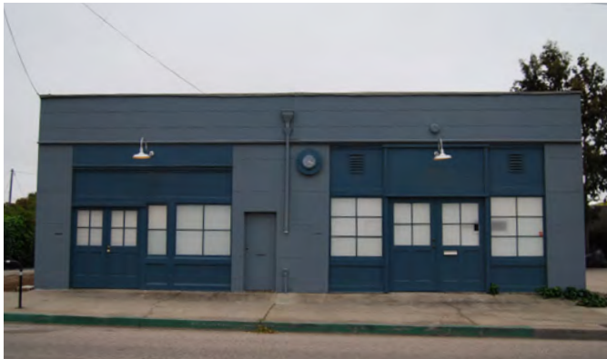
Example of a Maker Shopfront
