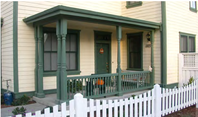
Example of an Engaged Porch
