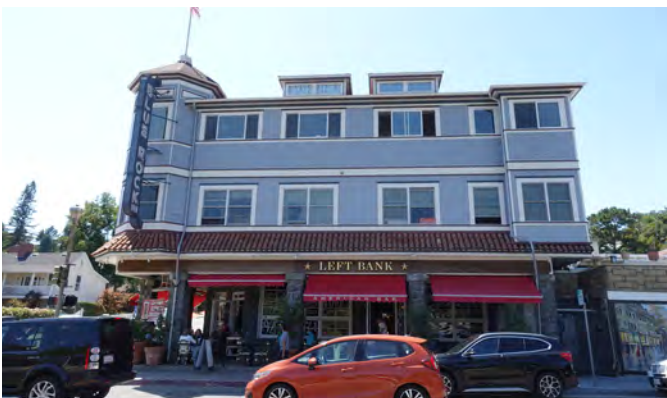
Example of Main Street Building
