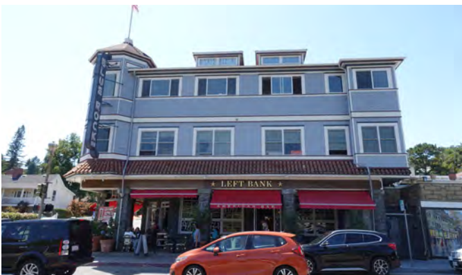
Example of Main Street Building
