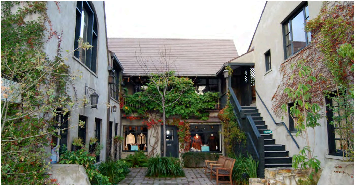
Example of a Forecourt with Shopfronts
