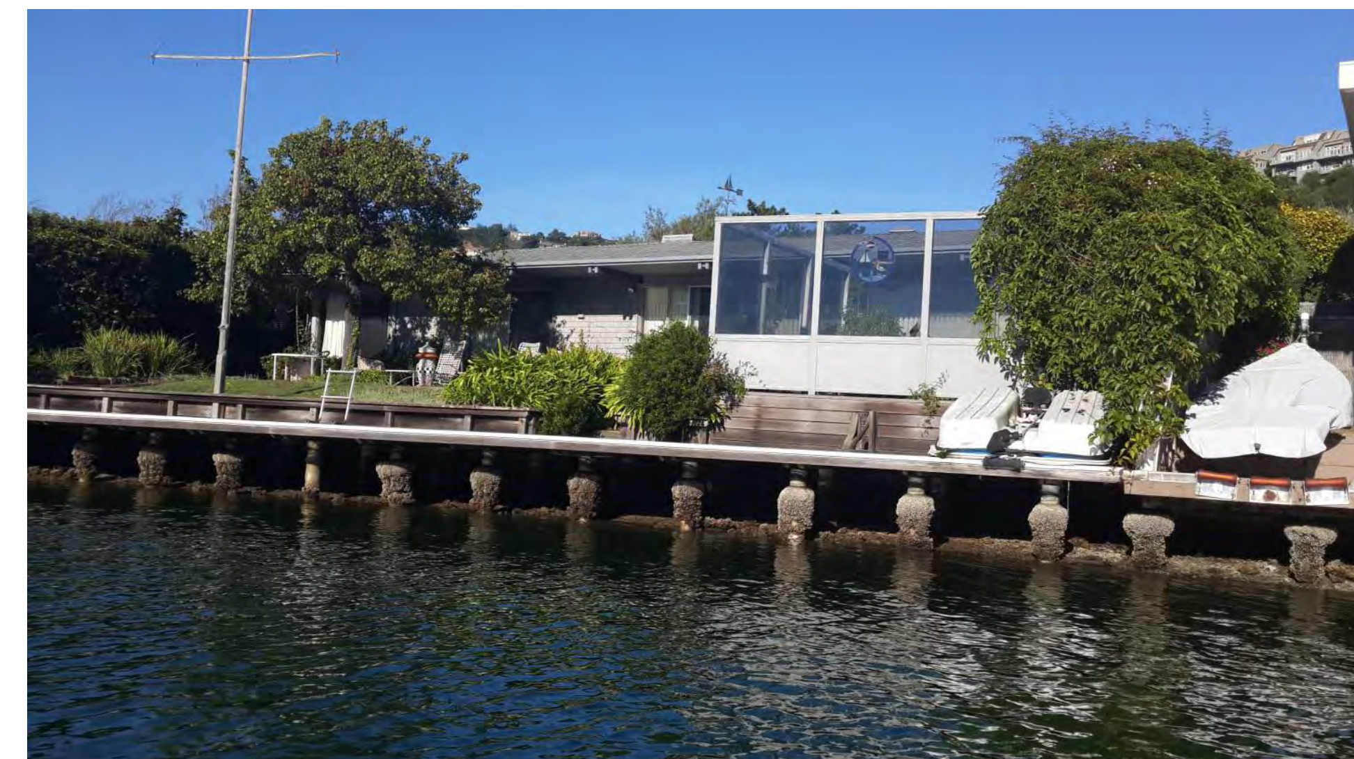
⑦ SITE PHOTO - REAR YARD FROM LAGOON 12" = 1'-0"
