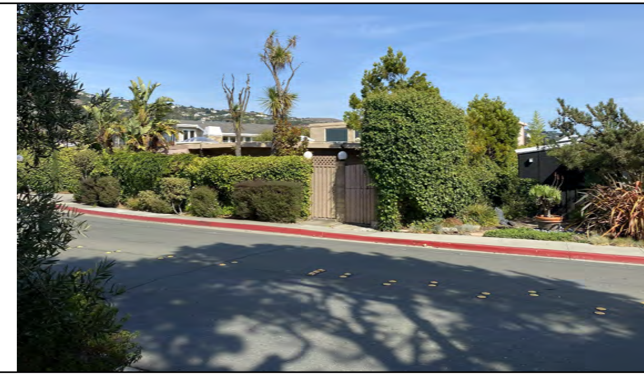
3. Front Facade image, looking East, with neighboring 160 San Rafael Ave. and 150 San Rafael Ave. Visible.
