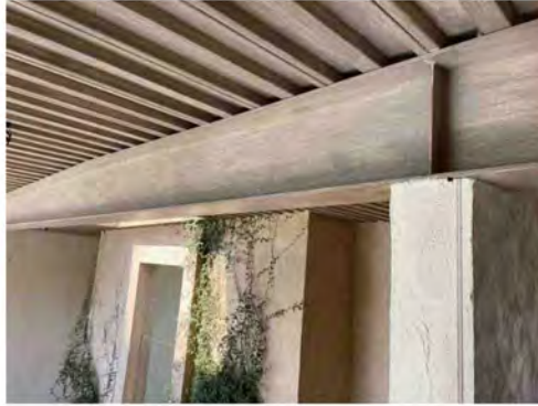
I beam and ceiling detail
