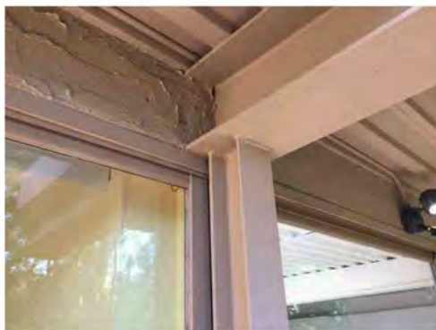
beam and window detail
