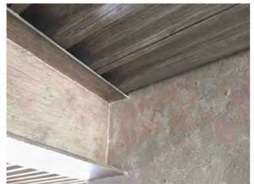
interior beam and ceiling
