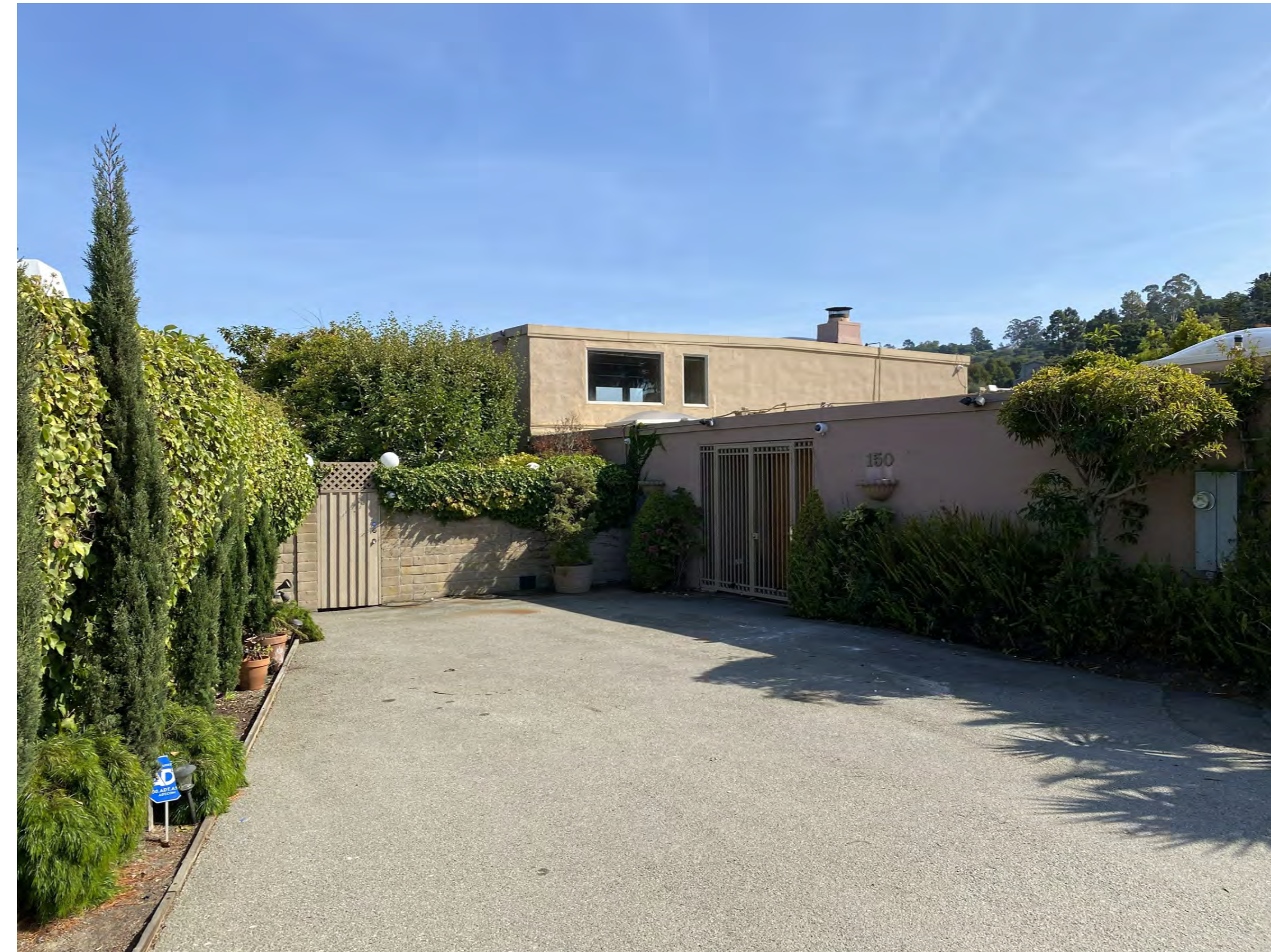
Photo 2: Existing Conditions Front Facade from outside edge of driveway. Showing Existing Entry Recess, Showing 2-Story portion to the rear Yard side of the lot, and the Driveway in the foreground.
