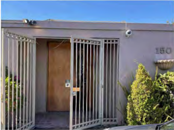
entry gate from driveway
