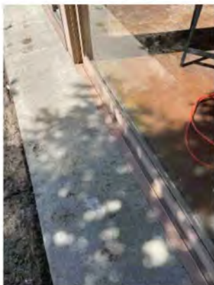
footing along living room
