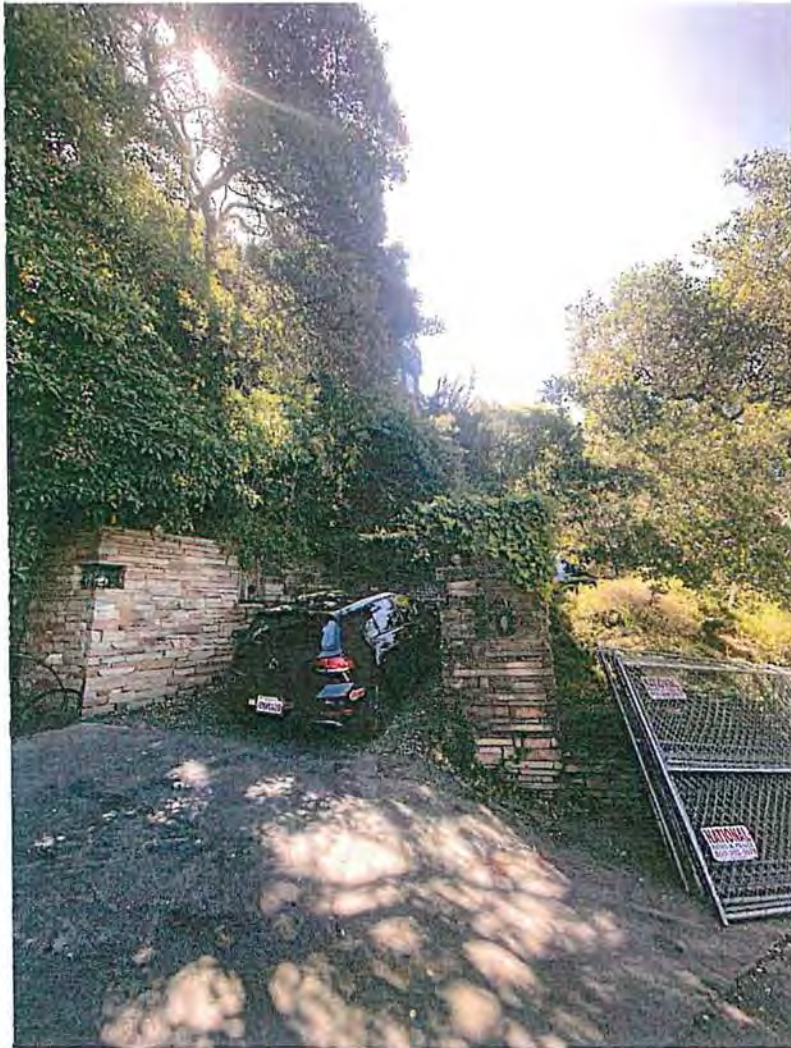
1. VIEW FROM CLIFF ROAD LOOKING UP DRIVEWAY
