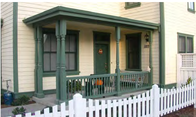
Example of an Engaged Porch
