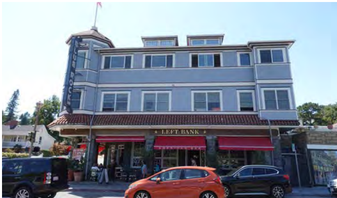
Example of Main Street Building
