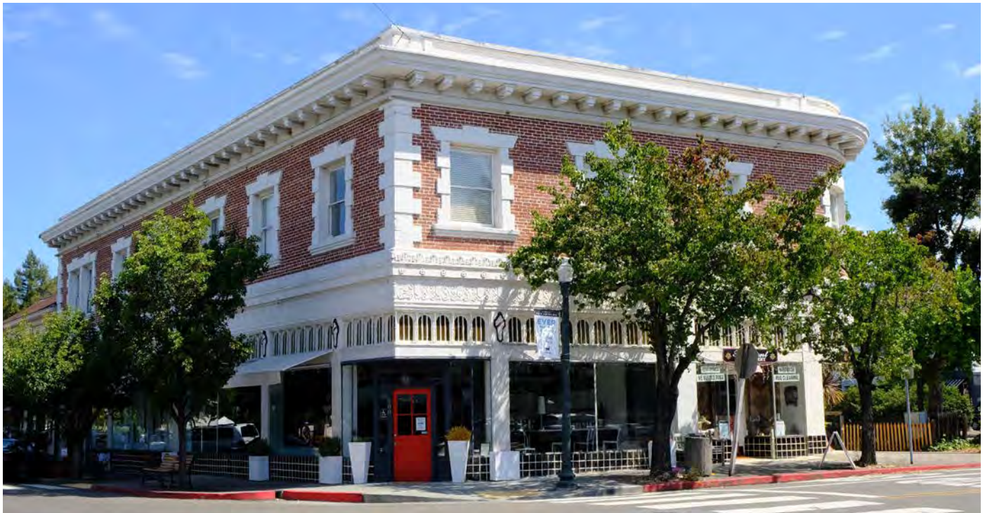
Example of Main Street Building
