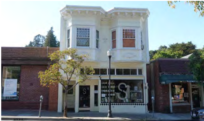
Example of Main Street Building
