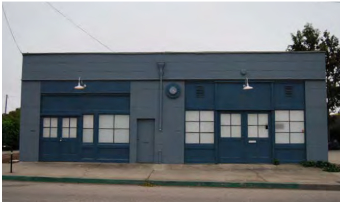
Example of a Maker Shopfront
