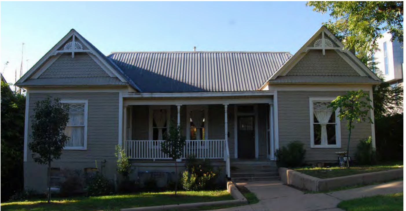
Example of an Engaged Porch
