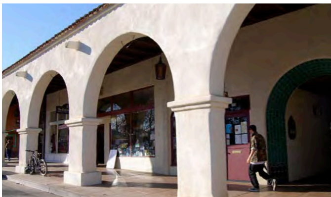
Example of a Gallery with shopfronts
