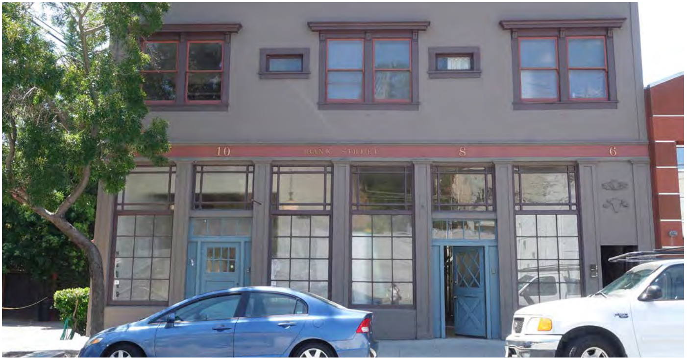
Example of a Maker Shopfront
