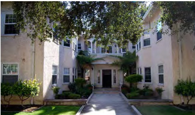
Example of Forecourt
