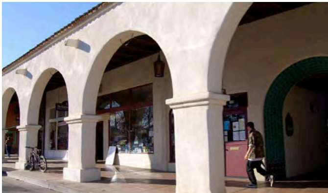
Example of a Gallery with shopfronts
