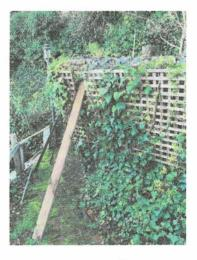
The retaining wall for the house just above the tum in the stairs is in very bad condition and has wooden supports to stop it from falling (photo right).
