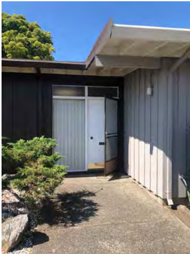
Fig.27 – 1-22 Mallard – Unit #18, front (north) entry
