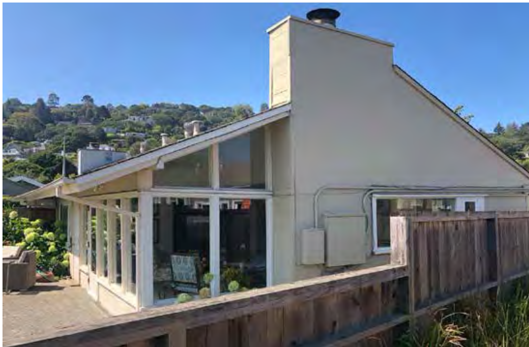
Fig.22 – 1-22 Mallard – Unit #11 Mallard, rear (north) and west side
