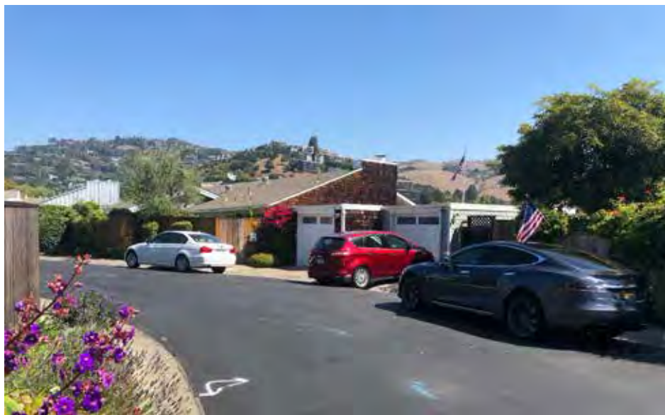
Fig.1A – 1-16 Mallard Rd. – View of lagoon side units, looking north
