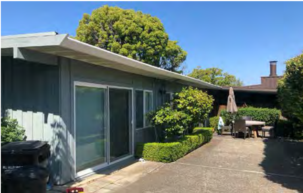
Fig.25 – 1-22 Mallard – Unit #17, front (north)
