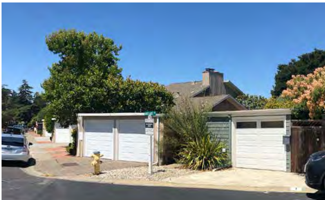
Fig.11 – 1-22 Mallard Rd. – View along west leg Mallard Rd. of lagoon side units, looking south
