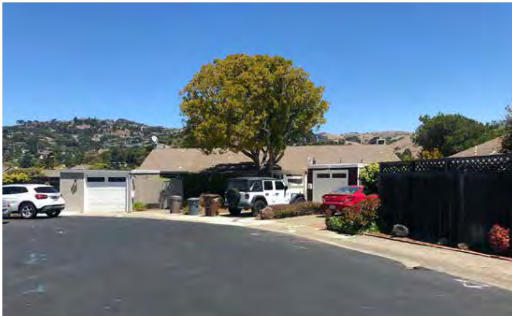
Fig.10 – 1-22 Mallard Rd. – View from north leg Mallard Rd. of lagoon side units 5-7 at point, looking north
