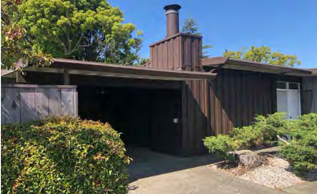
Fig.26 – 1-22 Mallard – Unit #18, front (north)
