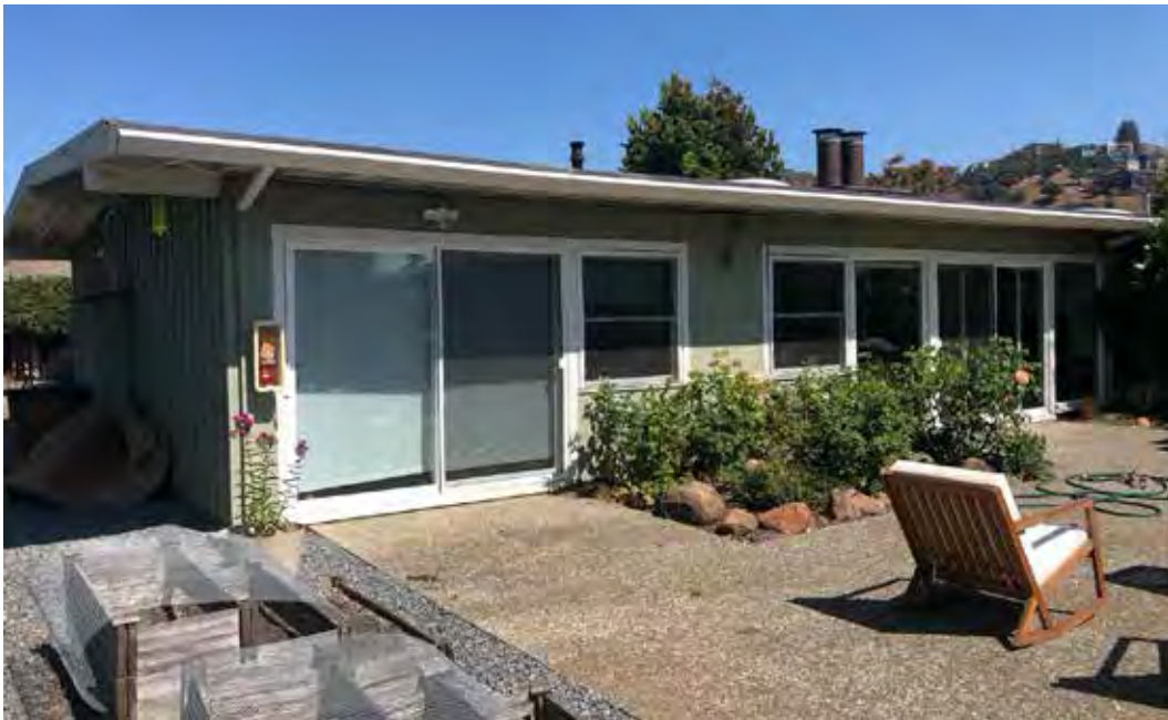
Fig.31 – 1-22 Mallard – Unit #22, south side and rear (east)
