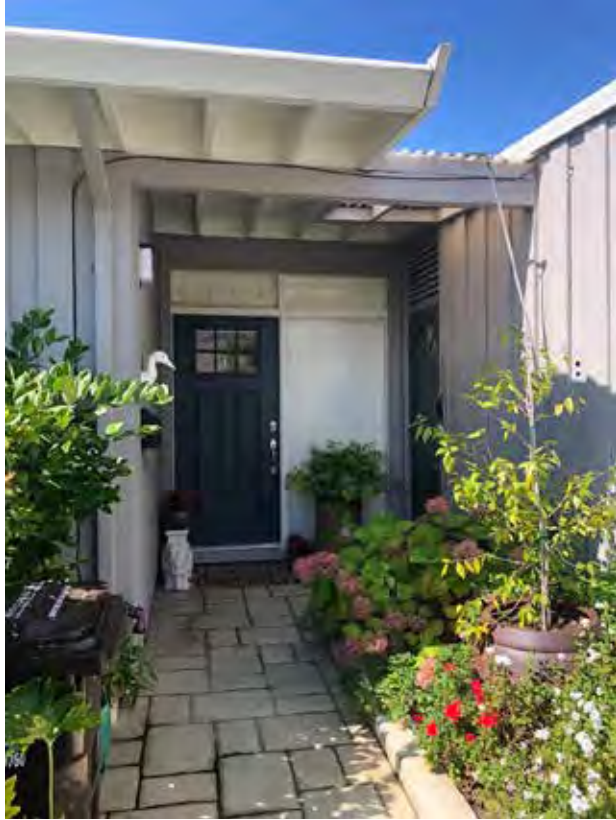
Fig.28 – 1-22 Mallard – Unit #19, front (north) entry
