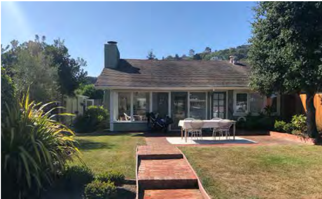
Fig.17 – 1-22 Mallard – Unit #2, rear(west)
