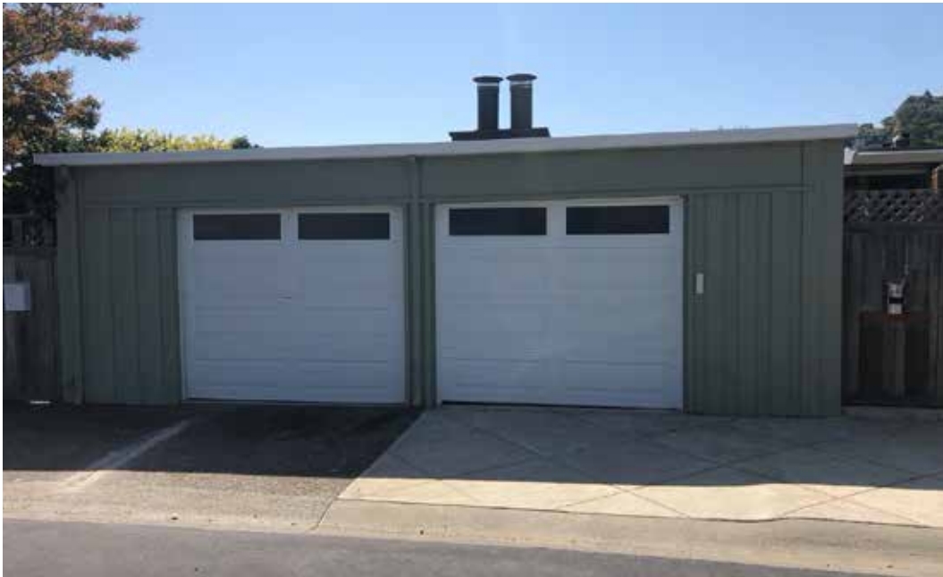
Fig.29 – 1-22 Mallard – Unit #21-22, garage fronts (west)
