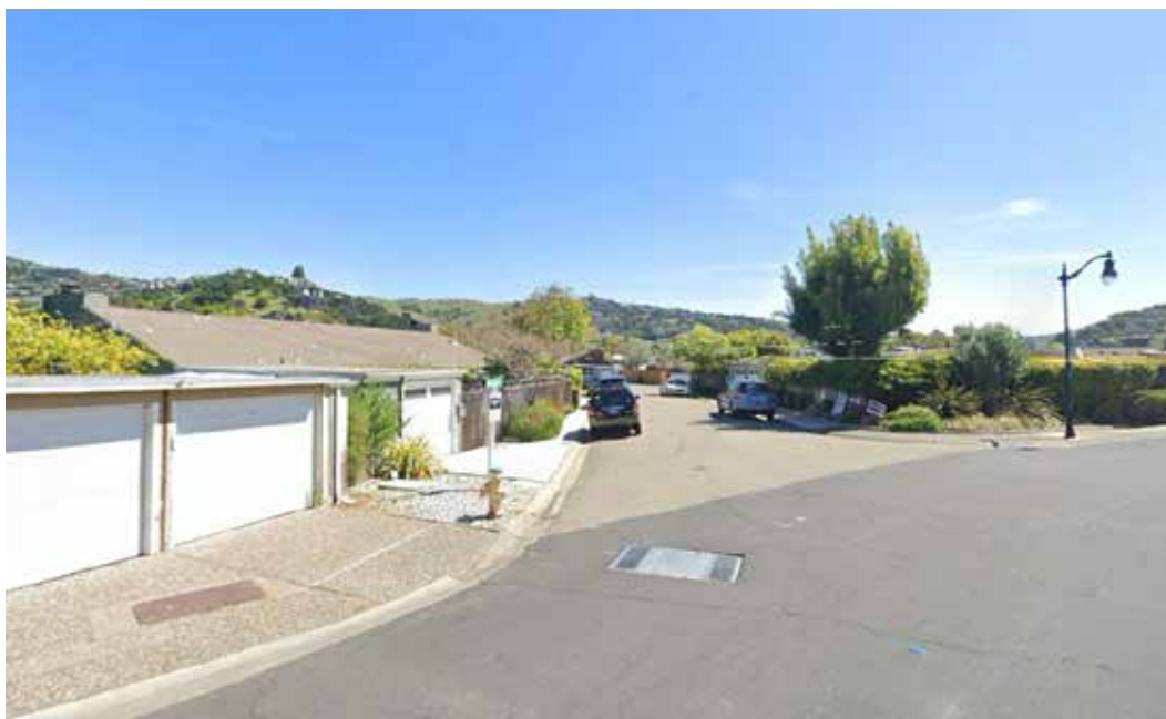
Fig.9 – 1-22 Mallard Rd. – View from Community Rd. into west leg Mallard Rd., looking north (google earth 2021)
