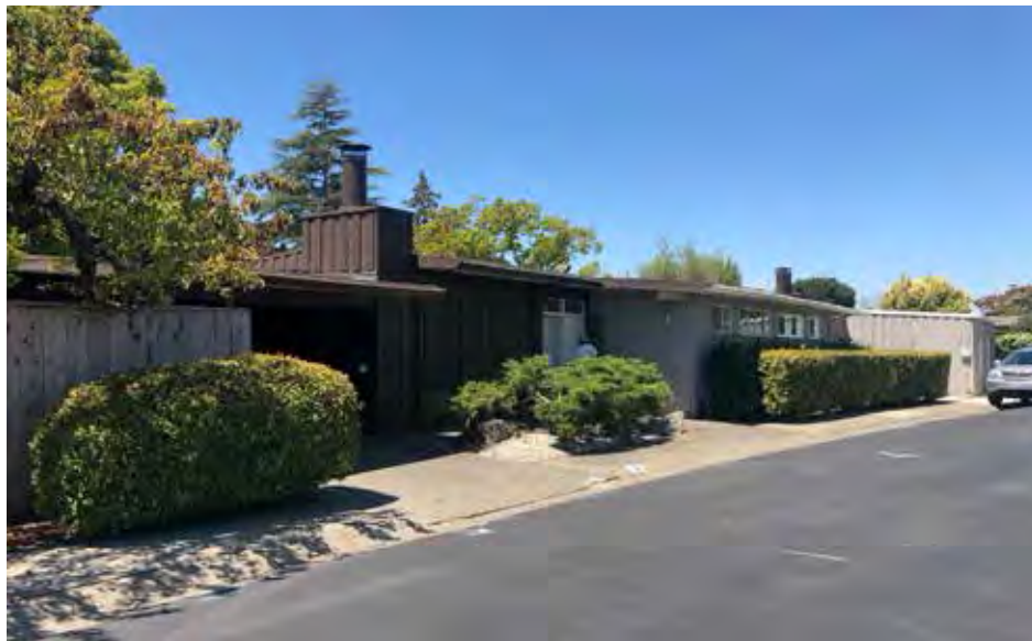
Fig.1B – 17-22 Mallard Rd. – View from north leg Mallard Rd., looking northeast
