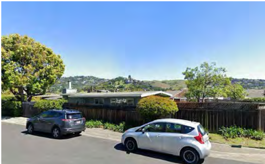
Fig.8 – 1-22 Mallard Rd. – View from Community Rd. of landside units, looking north (google earth 2021)
