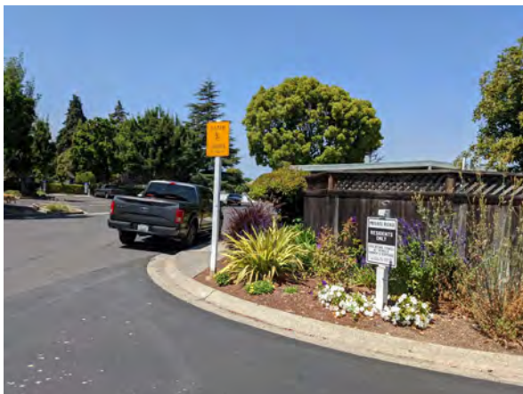
Intersections lack crosswalks and ADA-compliant ramps.
