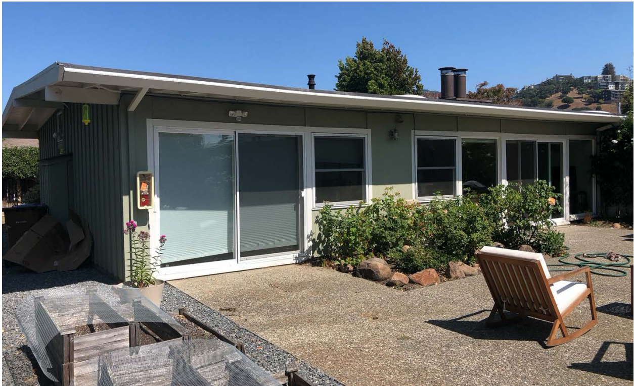
Fig.32 – 1-22 Mallard – Unit #22, south side and rear (east)
