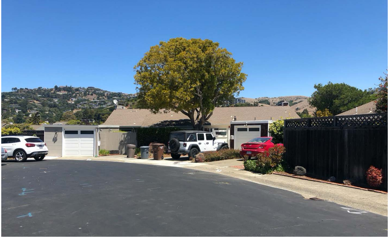
Fig.11 – 1-22 Mallard Rd. – View from north leg Mallard Rd. of lagoon side units 5-7 at point, looking north
