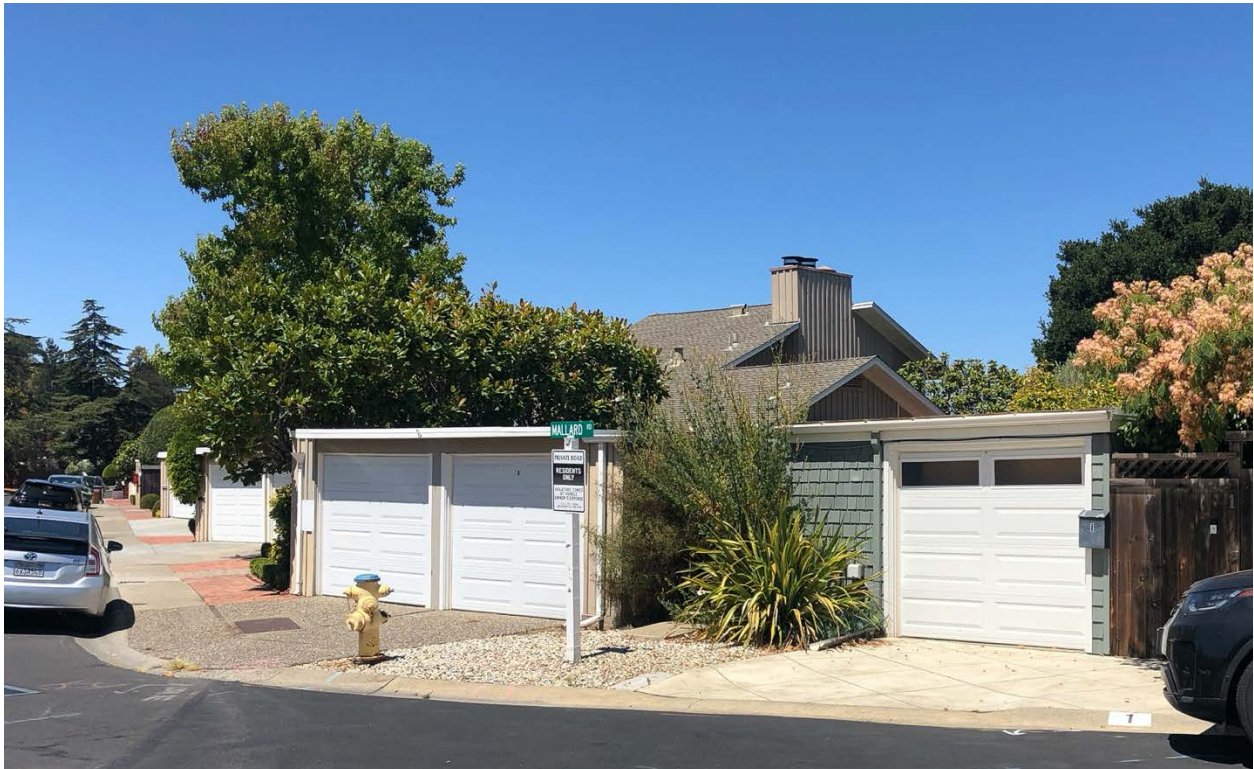
Fig.12 – 1-22 Mallard Rd. – View along west leg Mallard Rd. of lagoon side units, looking south
