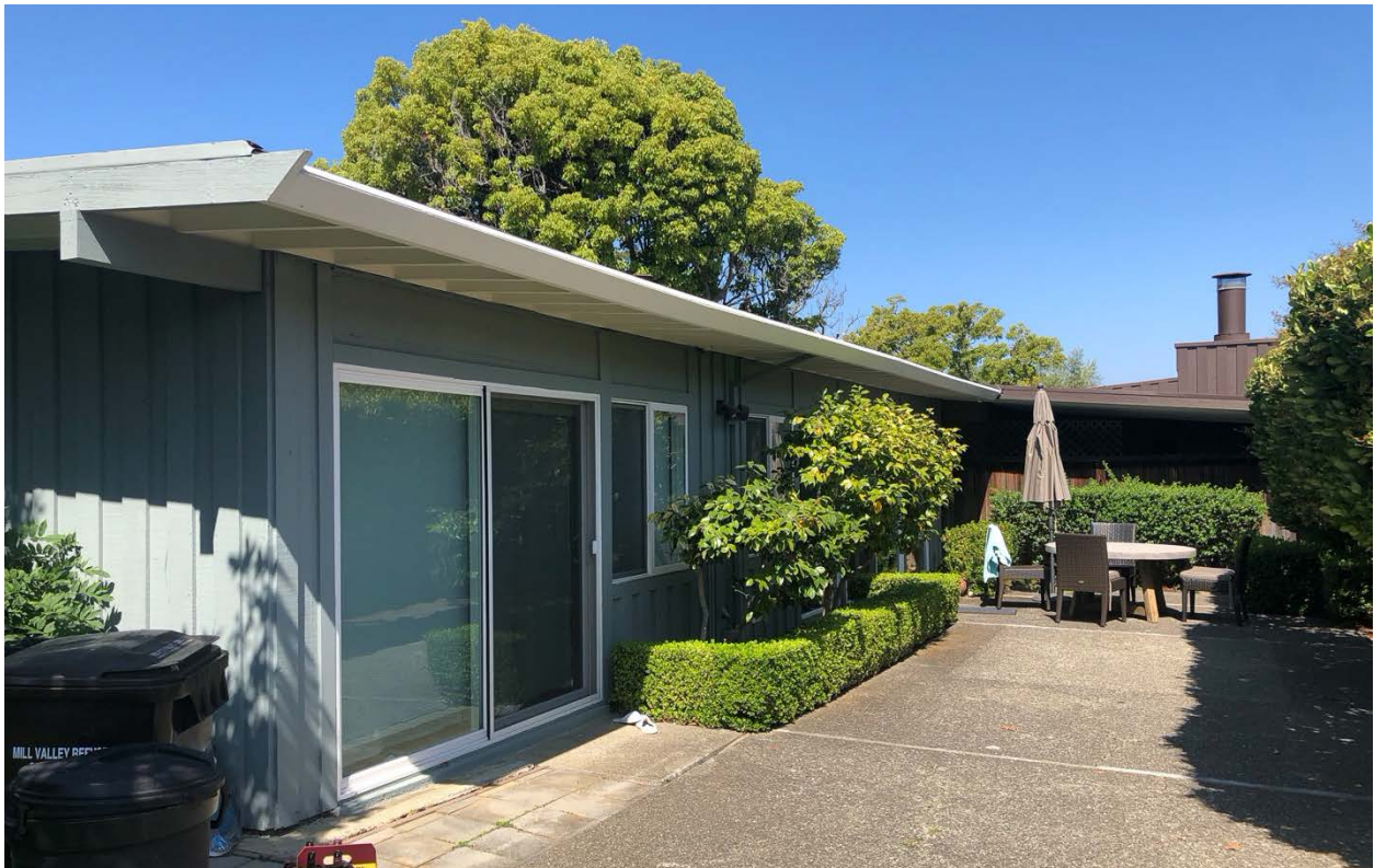
Fig.26 – 1-22 Mallard – Unit #17, front (north)
