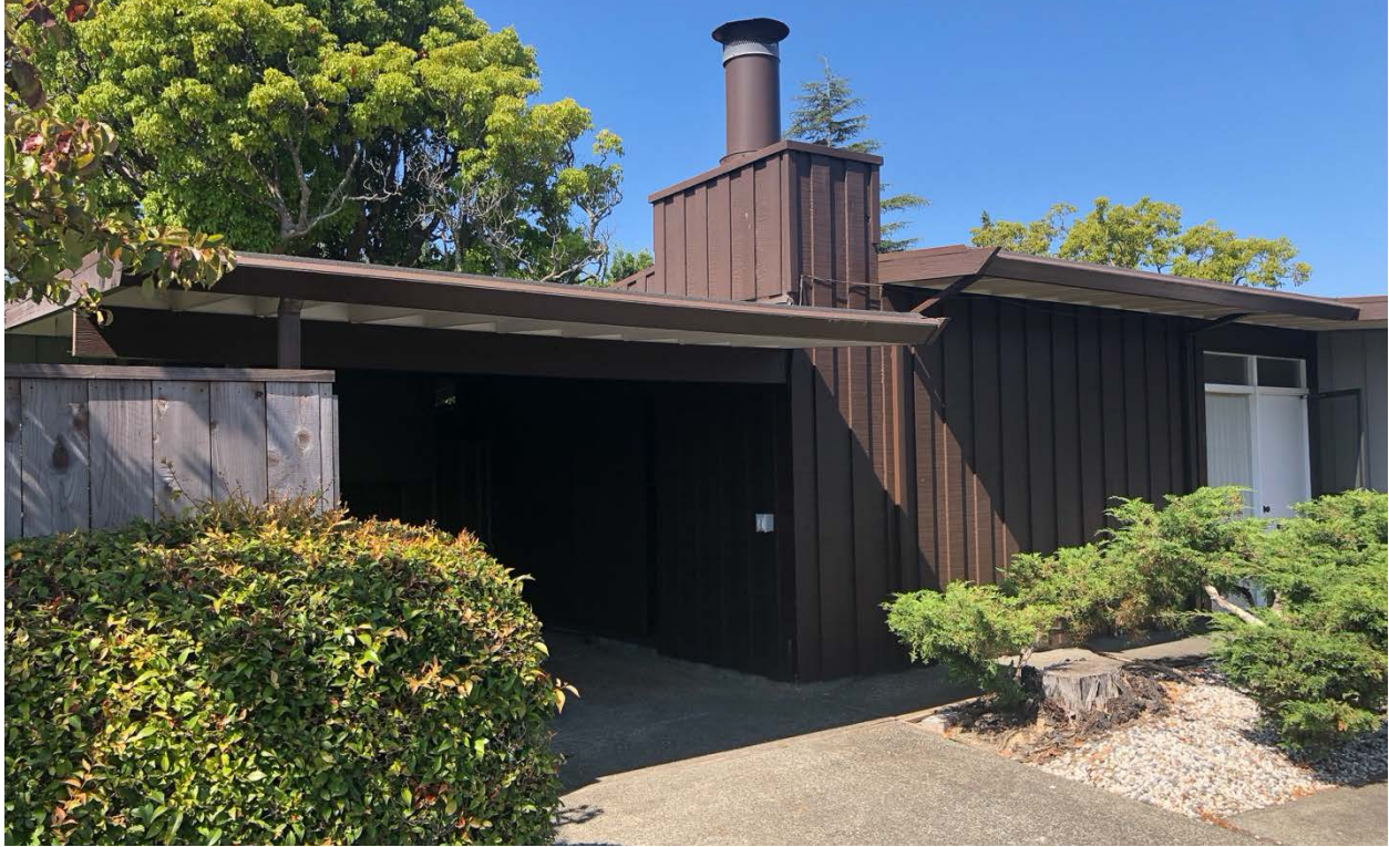
Fig.27 – 1-22 Mallard – Unit #18, front (north)
