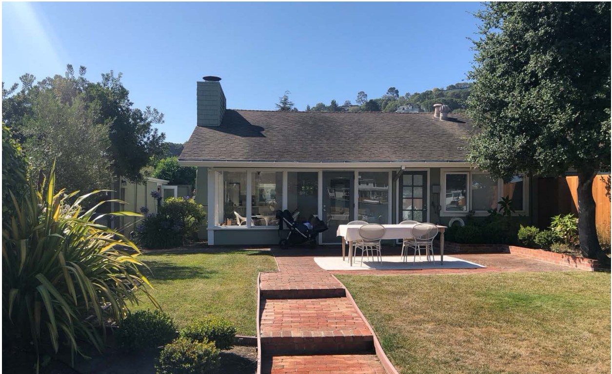
Fig.18 – 1-22 Mallard – Unit #2, rear(west)
