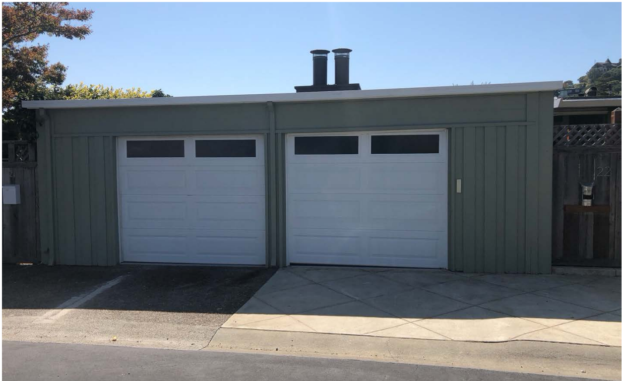
Fig.30 – 1-22 Mallard – Unit #21-22, garage fronts (west)
