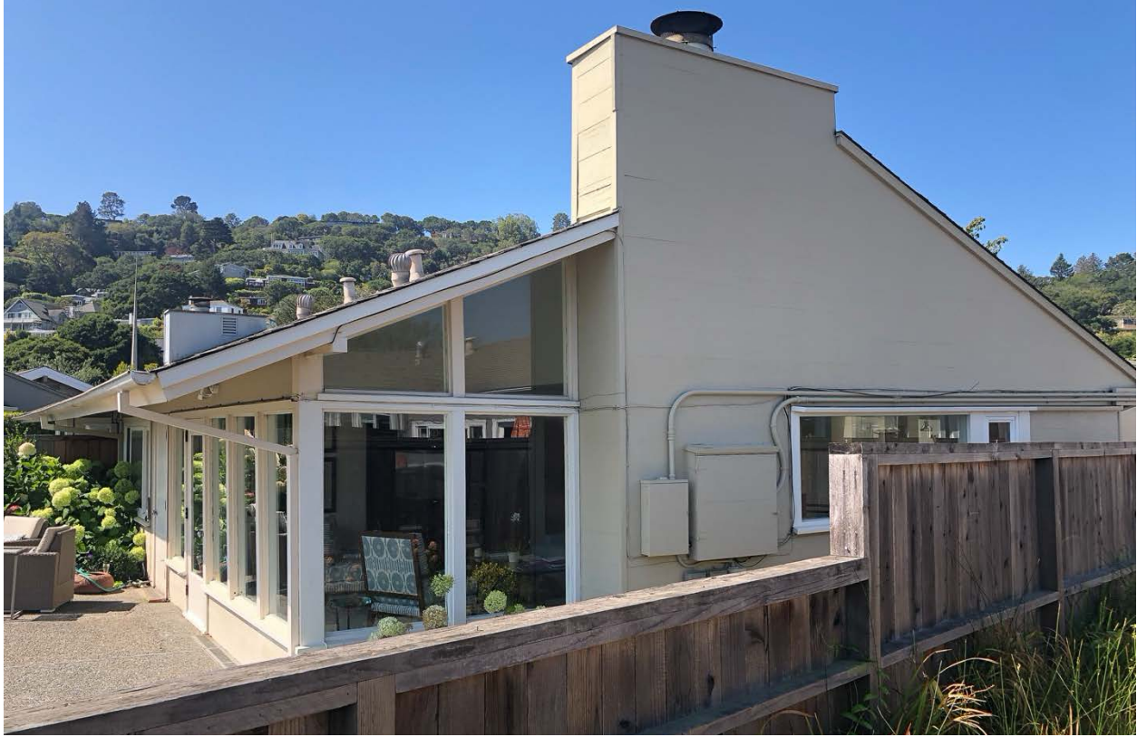
Fig.23 – 1-22 Mallard – Unit #11 Mallard, rear (north) and west side
