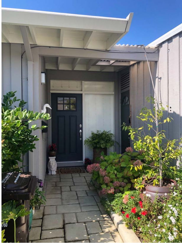
Fig.29 – 1-22 Mallard – Unit #19, front (north) entry
