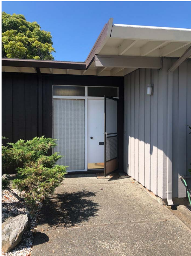
Fig.28 – 1-22 Mallard – Unit #18, front (north) entry
