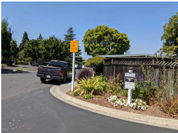
Intersections lack crosswalks and ADA-compliant ramps
