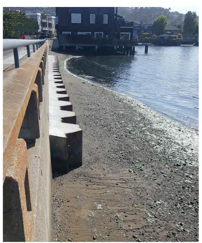
The left of the figure shows the existing seawall and hand rail. The 2019 sheet pile installation is located on the right along with the concrete connection to structurally support the existing seawall. New sheet piles along Beach Road that will be located bayside of the existing seawall will be installed in a similar manner.
