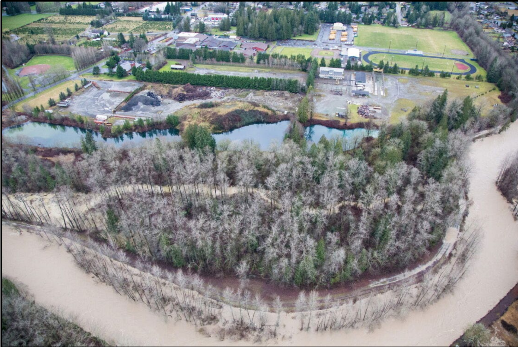
Tolt River flooding, January 2015
