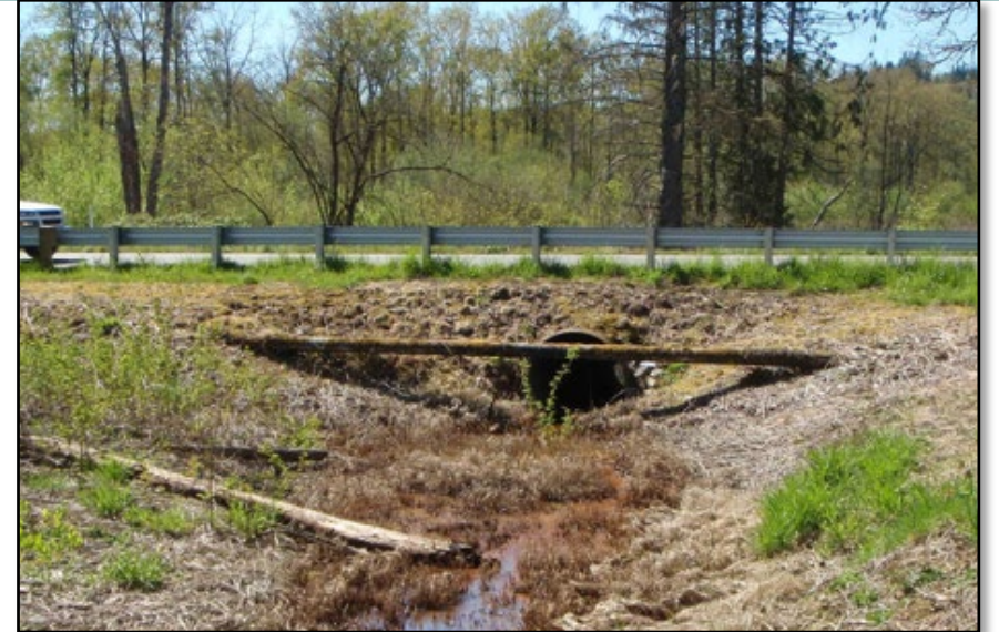
Existing culvert under SR 203
