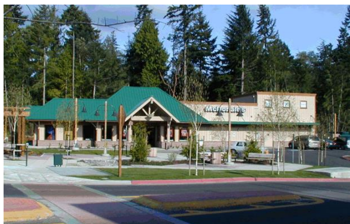
Figure 27. A combination of roof forms can be effective at reducing the scale of a building and adding visual interest.
