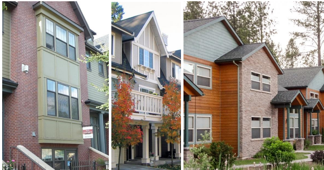
Figure 31. Details examples including bay windows and decorative materials (left image), balcony, decorative windows, and decorative roofline (middle image), and decorative materials and entry feature (right image)
