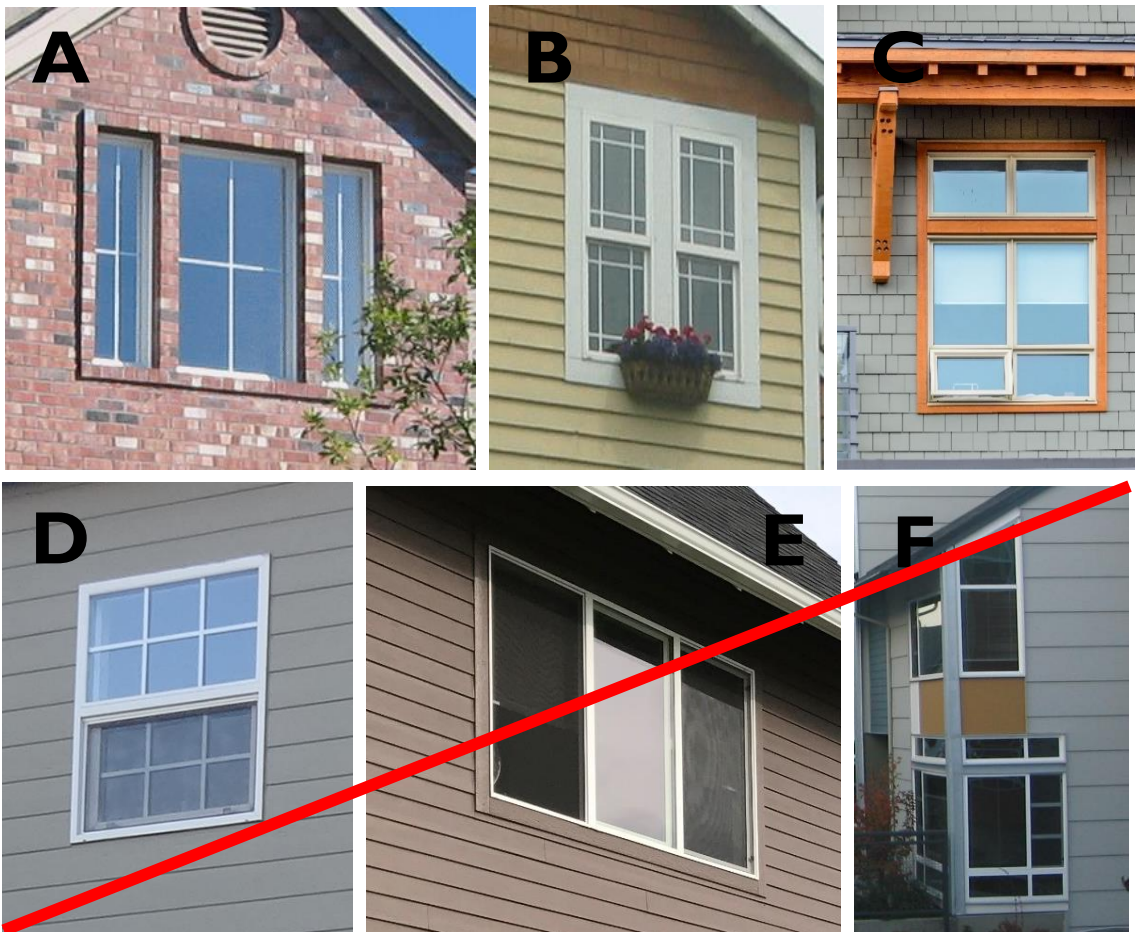
A: Grouped windows that are slightly recessed with brick trim. B & C: Windows with acceptable trim. D: Window does not contain sufficient trim. E: Trim does not contrast. F: Corner windows with insufficient trim.
