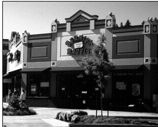
Figure 25. Overly ornate architectural styles and building details are discouraged.
