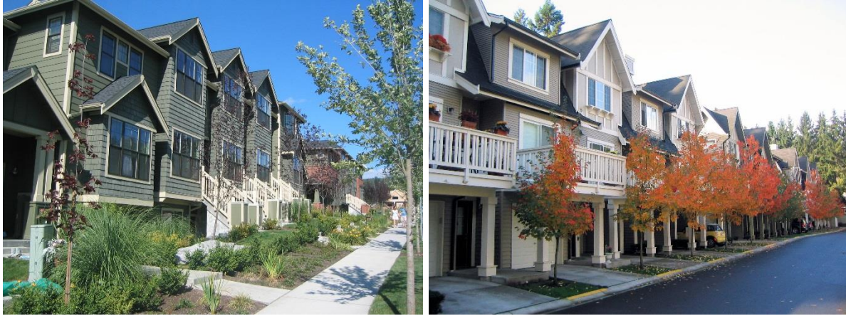
Left image – good: Roofline modulation, window design, elevated ground floor, and landscaping. Left image - room for improvement: Alternate siding and/or color could improve the design and reduce monotony. Right image – good: Design with balcony in front softens the rest of the façade, roofline variation, siding style. This design with garages/driveways is appropriate along internal drives, but not adjacent to public streets.
