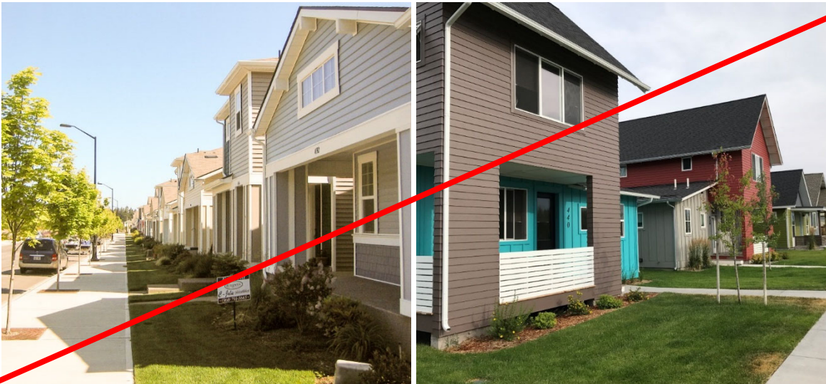
Above: Top-heavy and flat facades with cave-like inward modulations.
