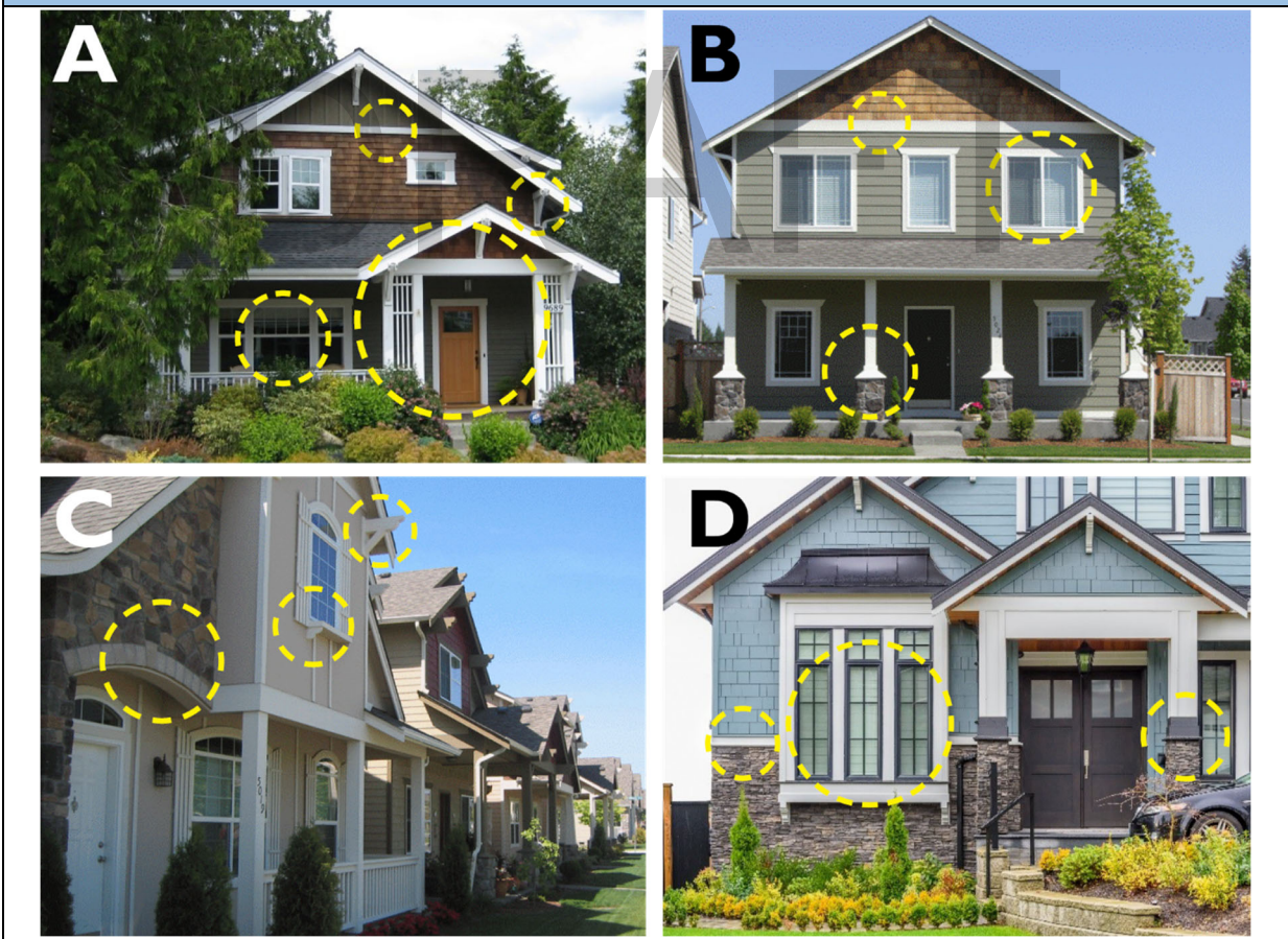
A: Decorative window framing, decorative entry design, roof brackets, decorative/contrasting siding materials. B: Decorative porch supports, window treatment, contrasting siding color and materials. C: Decorative building materials, feature door/entry, decorative window framing, roof brackets. D: Decorative building materials, bay window, decorative porch supports.
