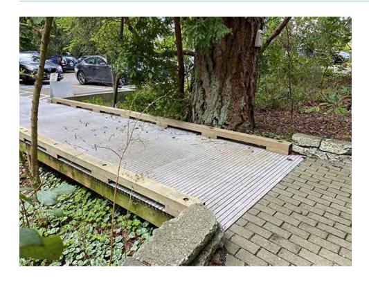
Left: Floating walkway constructed next to large Douglas-fir at Kruckeberg Botanical Garden in Shoreline, WA. Supports are set at least 8 feet apart, using long timbers to minimize root disturbance. Openings between deck boards allow rainwater to flow to roots.
