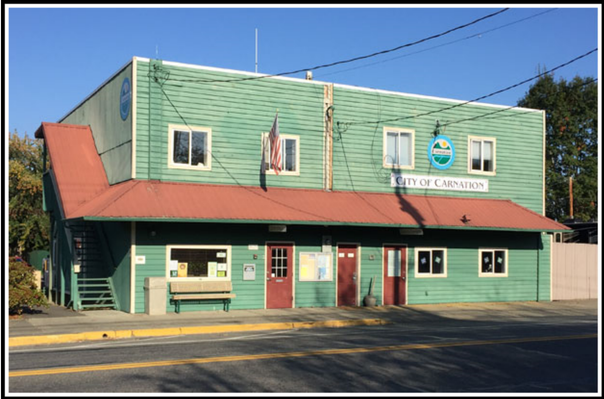
Photo 1 – East Exterior View of Building
