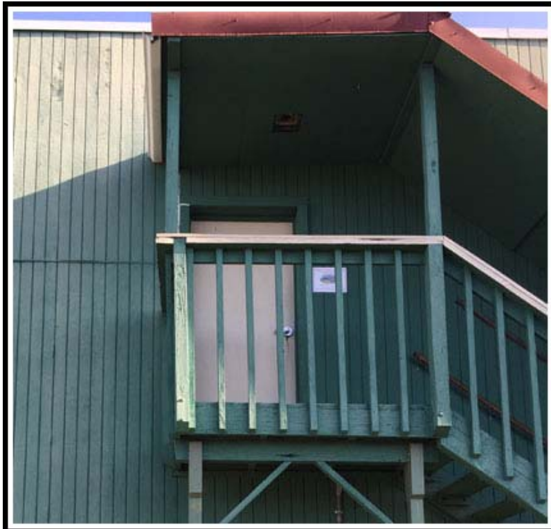
Photo 4 – South Exterior Second Floor Stair Landing
