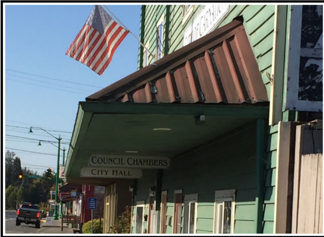
Photo 7 – Exterior Awning on East Side of Building
