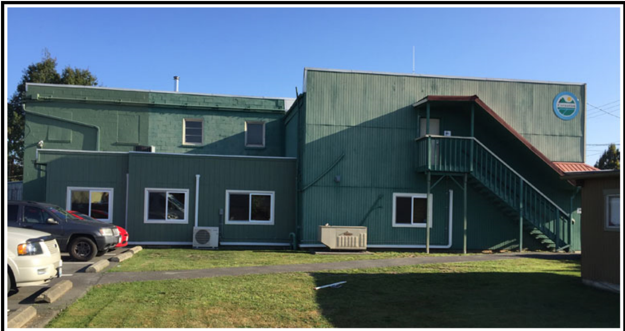
Photo 2 – South Exterior View of Building
