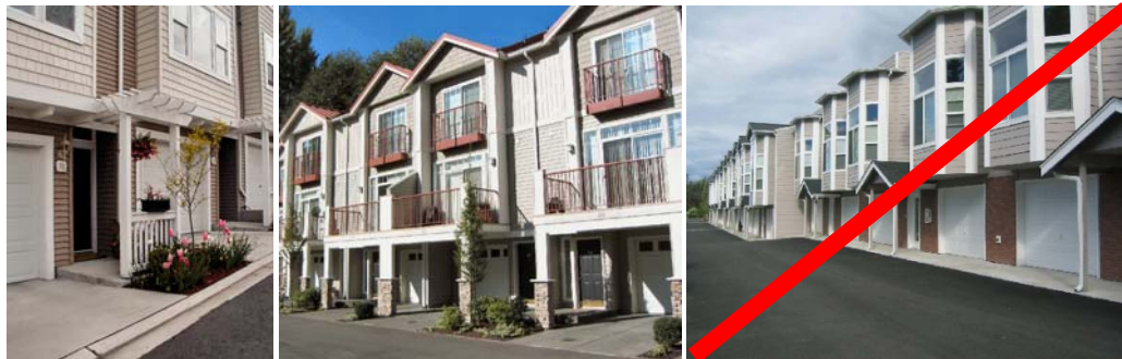
Figure 35._Acceptable and unacceptable examples of garage/entry configurations. The left example features a landscaped area and a trellis to highlight the entry. In the middle image, the balconies and landscaped areas deemphasize the garage. In the right image, the lack of landscaping near the entries would not be allowed (where this is the primary pedestrian entry to the unit).
