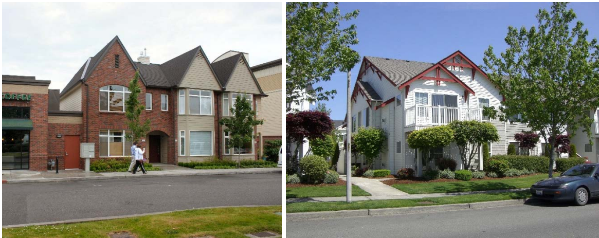
Left image – good: Roofline and facade modulation, windows and entry design, materials, front landscaping. Left image - room for improvement: Wider front setback would be good particularly if ground floor is not elevated. Right image – good: Modest scale, front landscaping, and roofline design details. Right image – room for improvement: Greater façade color variation.
