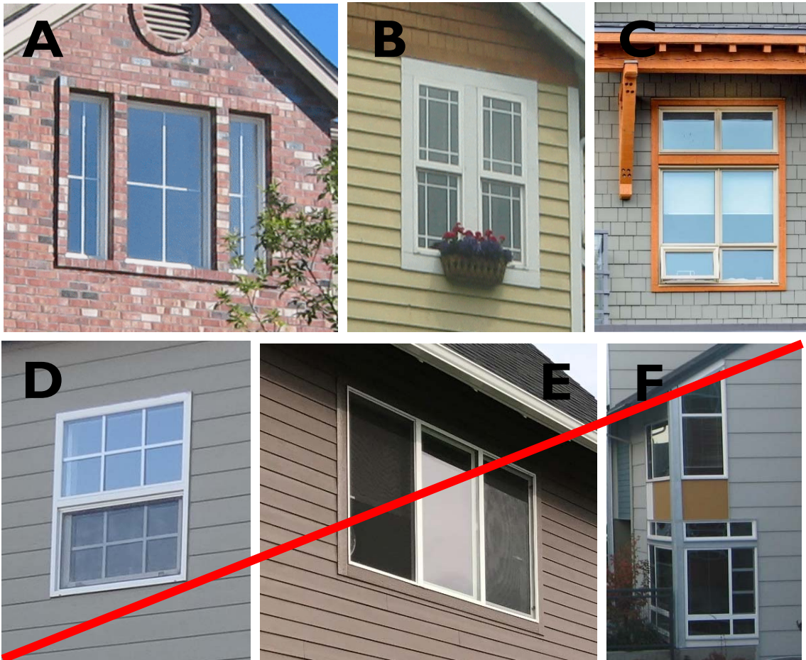
A: Grouped windows that are slightly recessed with brick trim. B & C: Windows with acceptable trim. D: Window does not contain sufficient trim. E: Trim does not contrast. F: Corner windows with insufficient trim.
