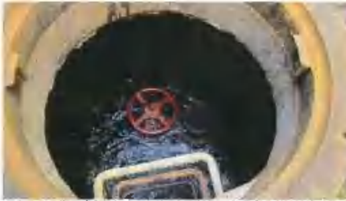
Spring Collection: (L) Inside of overflow vault; overflow through standpipe to creek. Sump in vault should keep water level down; no sump pump. (R) A pump in the chlorination building draws a stream of water from this structure (through the PVC pipe); chlorine is injected and mixed inline; injection point is in separate vault downstream.
