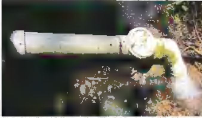
Spring Collection: (L) Overflow pipe with irrigation flapper valve. (R) Vault contains magmeter to measure flow to town and injection point for chlorination.
