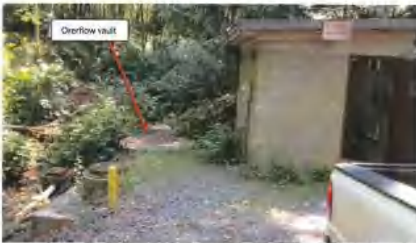
Spring and Chlorination Building Overview: View of chlorination building, looking back towards springs. Overflow vault on far left; overflows to creek.
