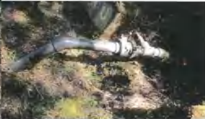
Horizontal Wellpoints: (L) and (R) Close up of well point piping. Sample bar shown on well in left.
