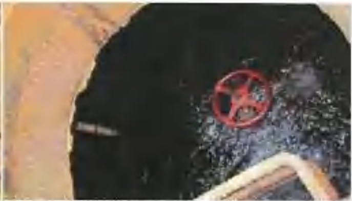
Spring Collection: (L) Inside of overflow vault; overflow through standpipe to creek. Sump in vault should keep water level down; no sump pump. (R) A pump in the chlorination building draws a stream of water from this structure (through the PVC pipe); chlorine is injected and mixed inline; injection point is in separate vault downstream.
