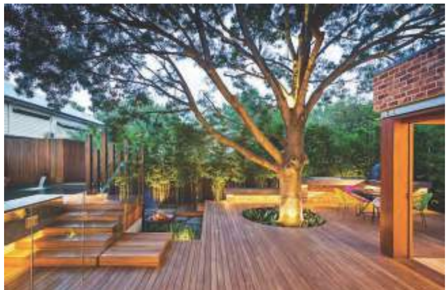
Right: Floating deck built around tree, featured on nextluxury.com. Used only as example for reference. No copyright infringement intended.
