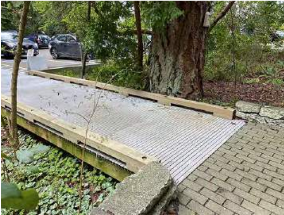
Left: Floating walkway constructed next to large Douglas-fir at Kruckeberg Botanical Garden in Shoreline, WA. Supports are set at least 8 feet apart, using long timbers to minimize root disturbance. Openings between deck boards allow rainwater to flow to roots.
