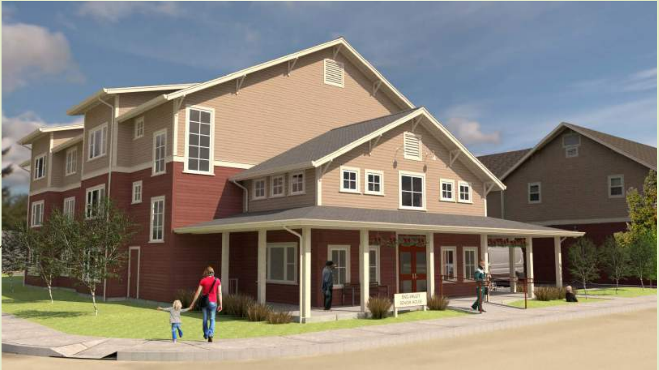
View of Front Porch from Stephens Avenue
