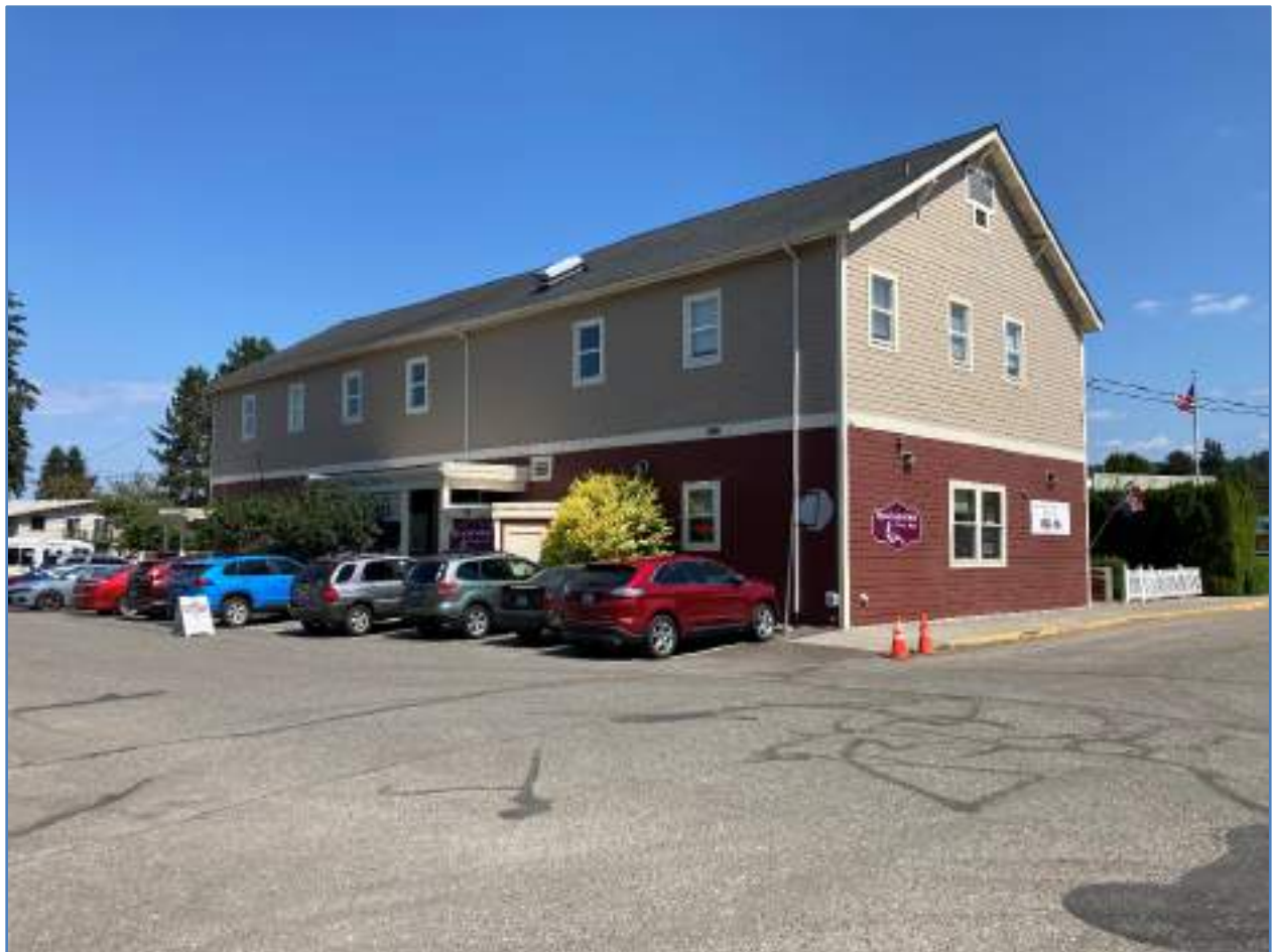
Figure 8. Existing Sno-Valley Senior Center (SVSC) building (formerly IOOF lodge), view NE.
