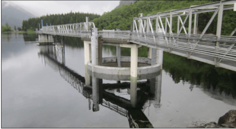
Tolt River reservoir and Morning Glory spillway. Photo: City of Seattle
