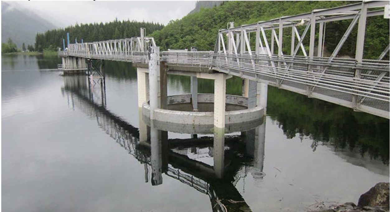
Tolt Reservoir and Morning Glory Spillway. From Seattle.gov
