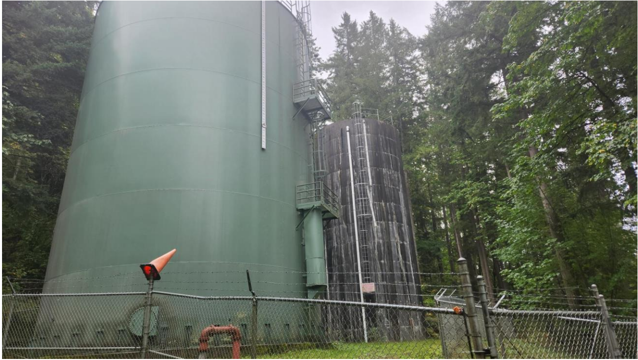
3. Looking NE toward water tank from proposed tower and lease area
