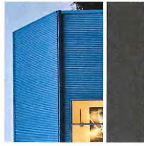
7 A-5.2 CORR. METAL SIDING/ROOF BARRIDGE "CHARCOAL GREY"
