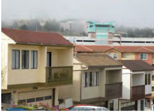
The parking structure serving the Colma BART Station seen in the distance, over homes in Colma's Sterling Park neighborhood. Colma residents can easily access both the Colma BART Station and the South San Francisco BART Station. It is anticipated that parcels near these stations will see high density, mixed use development.
