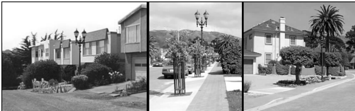
The utility undergrounding project in Sterling Park (under construction, left) has resulted in the creation of a handsome streetscape (middle and right).
