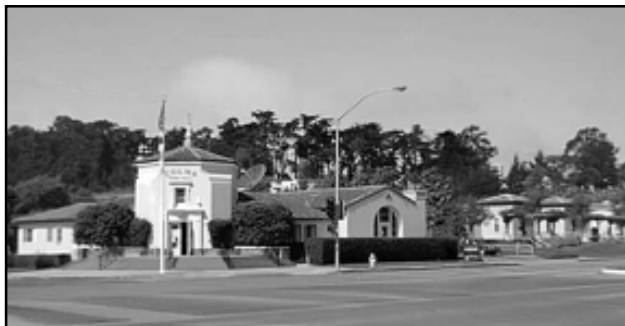
Colma's government offices. The Spanish-style architecture of Town Hall provided the inspiration for Colma's design guidelines.
