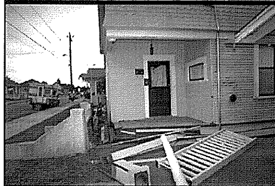
In earthquakes, unreinforced masonry buildings (top) are particularly vulnerable. Wood-frame buildings generally perform well, although an earthquake's lateral force may cause structures to separate from their foundations (the house in the bottom photo was originally positioned next to the stairway).
