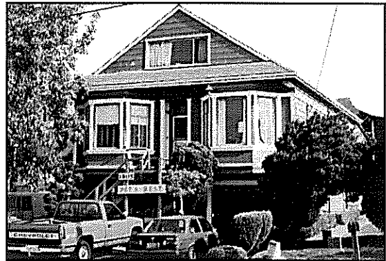
F. Pet's Rest Cemetery Office 1905 Hillside Boulevard Rating: Historic Resource
