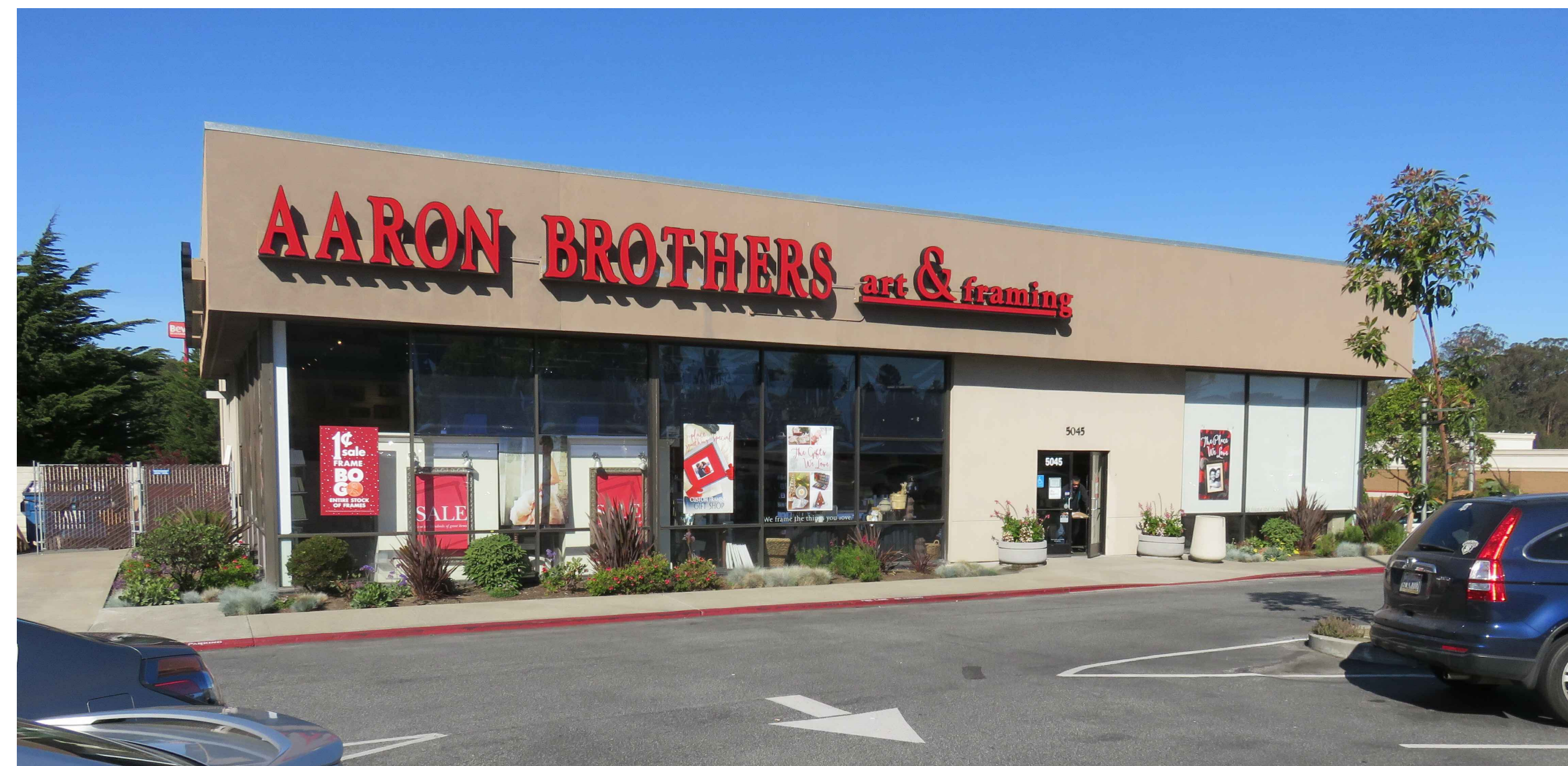
EXISTING CONDITIONS - NORTH ELEVATION
