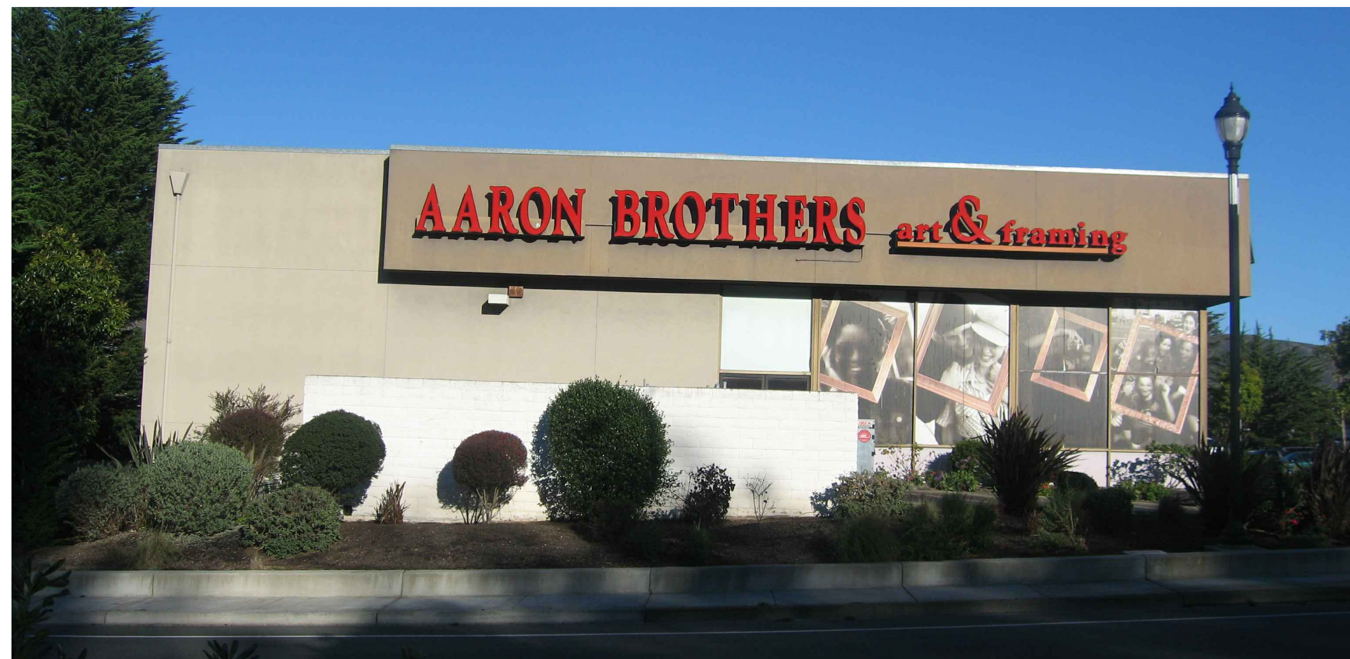
EXISTING CONDITIONS - WEST ELEVATION
