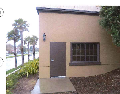
3 EXISTING 1ST FLOOR REAR DOOR
