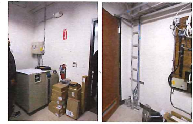
4A NORTH WALL PHOTO ELEV. NTS
