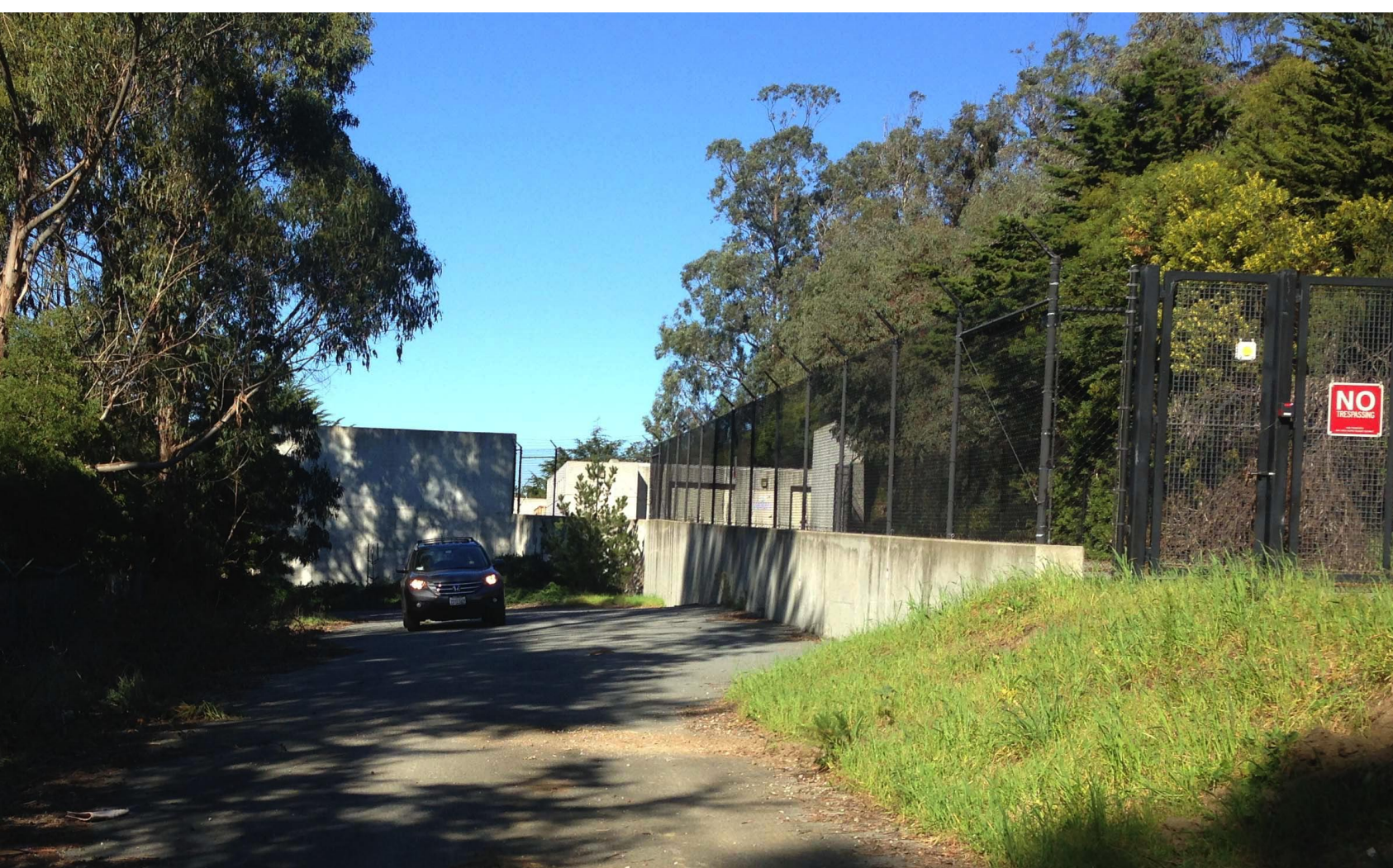
6 A-0.3 VIEW FROM BART ACCESS ROAD
