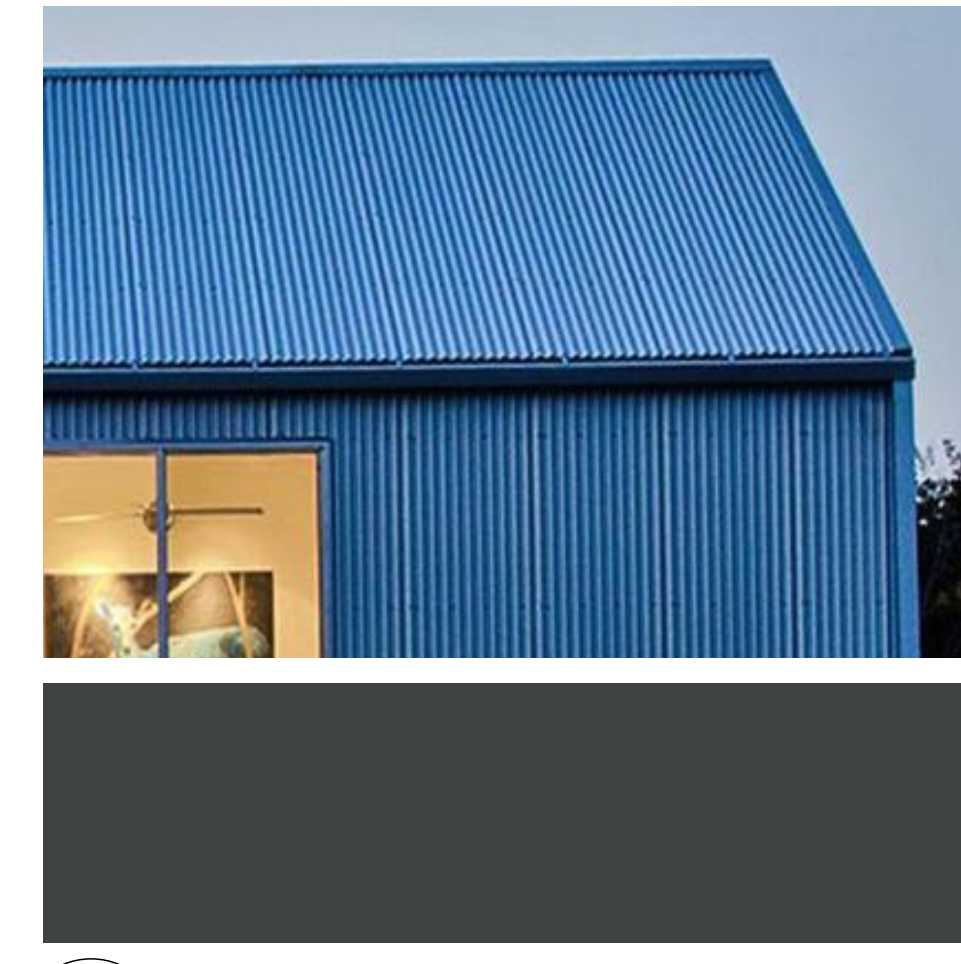
7 A-5.2 CORR. METAL SIDING/ROOF BARRIDGE "CHARCOAL GREY"
