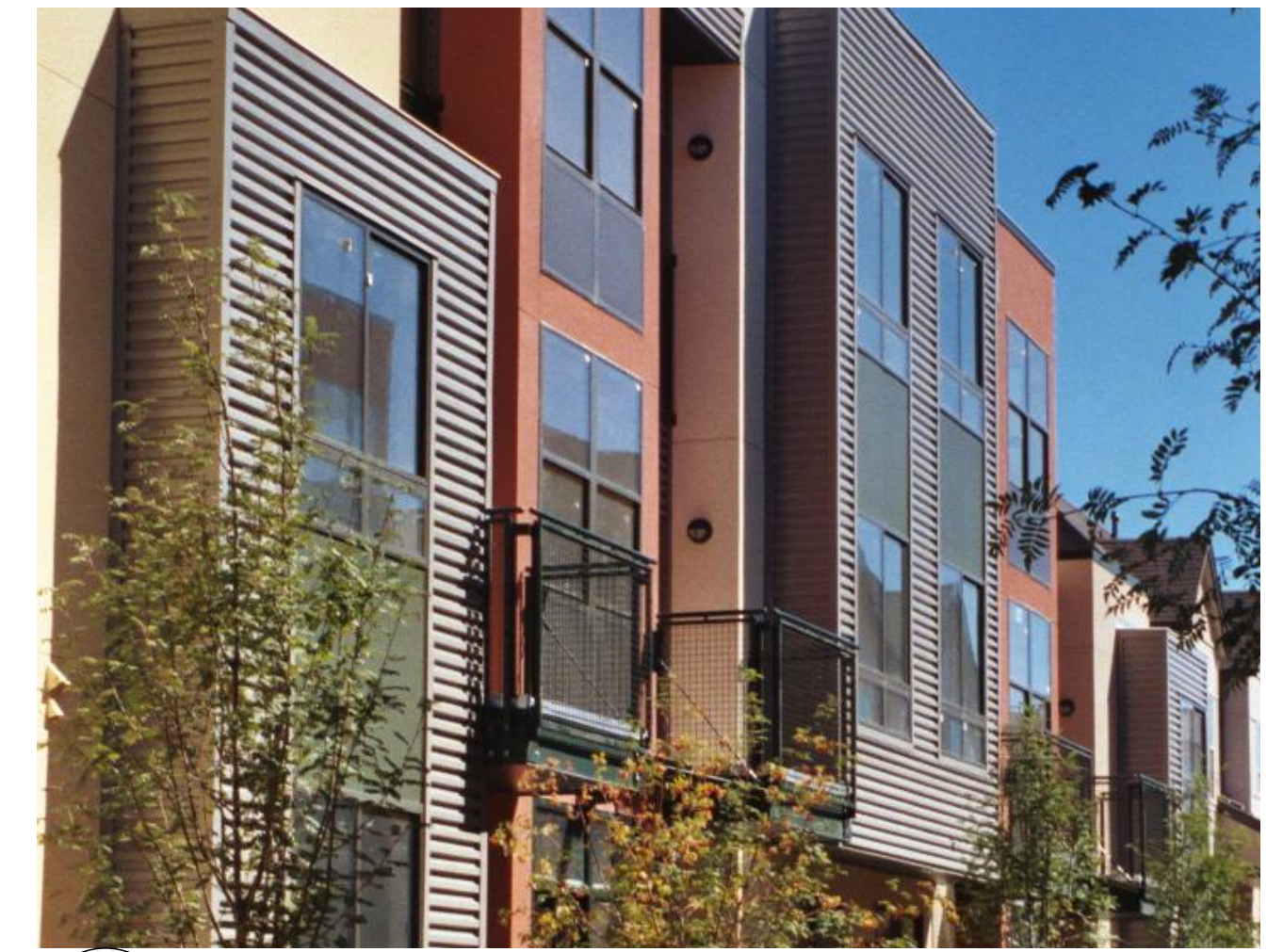
2 A-5.2 FIBER CEMENT PANEL AT WINDOW
