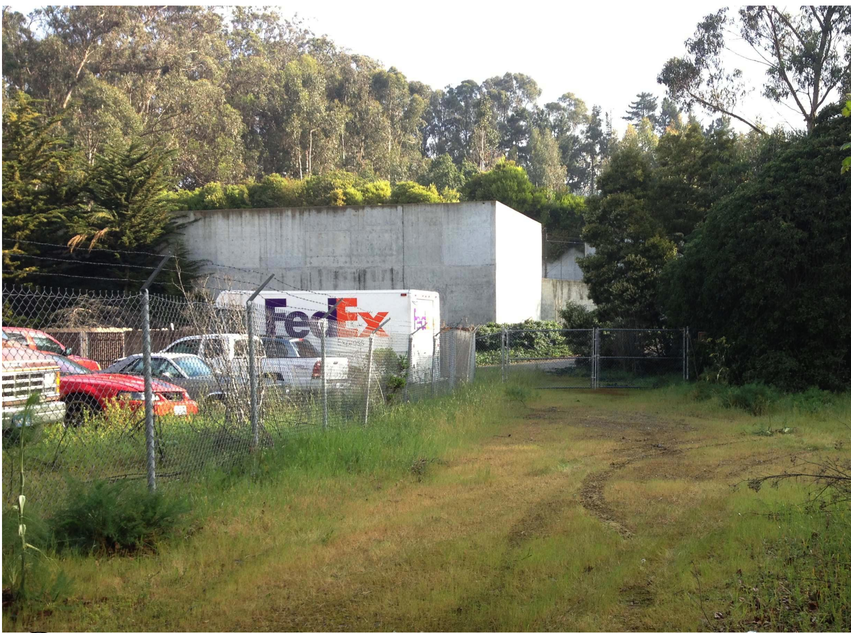
4 A-0.3 VIEW TO BART STRUCTURE
