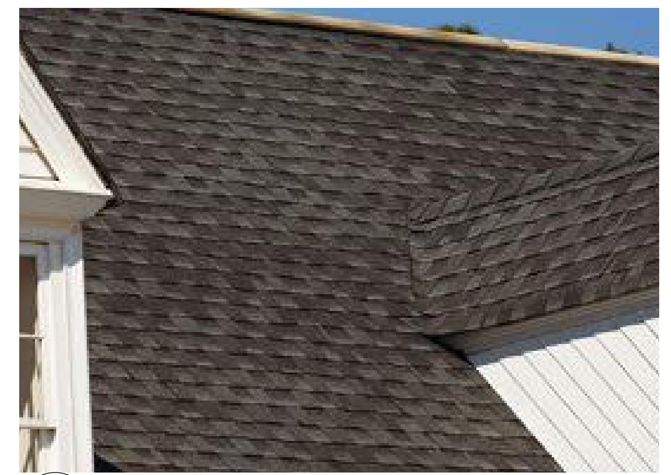
1 A-5.2 COMPOSITION SHINGLE ROOF
