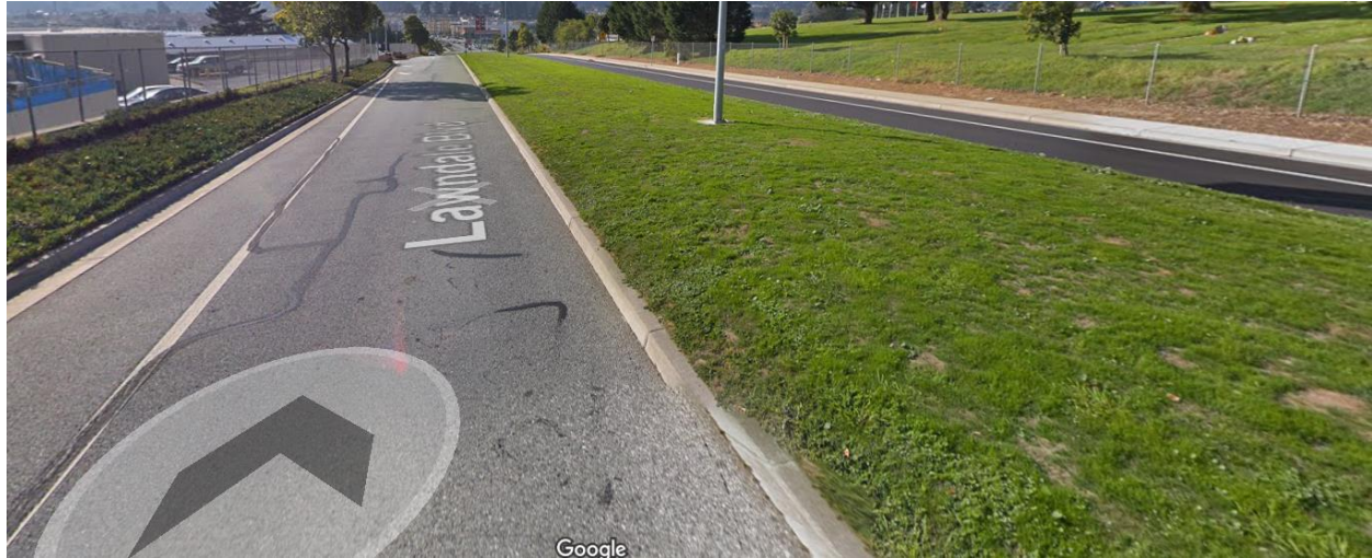
Figure 60: Existing Conditions at Lawndale Boulevard
