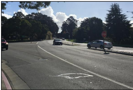
Figure 40: Location along Mission Road in Need of Traffic Control.
