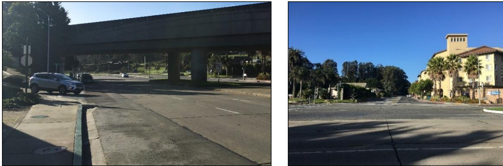
Figure 48: Existing Conditions at El Camino Real/F Street Intersection.
