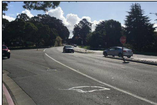
Figure 31: Location along Mission Road In Need of Traffic Control.
