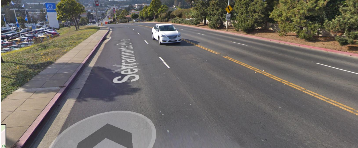
Figure 58: Existing Conditions on Serramonte Boulevard
