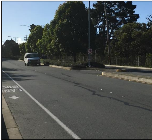
Left-in only driveway access (vi)
