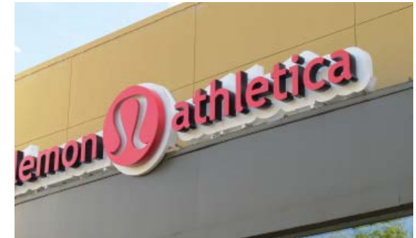
EXAMPLE: SIGNAGE SUPPORTED FROM BELOW
