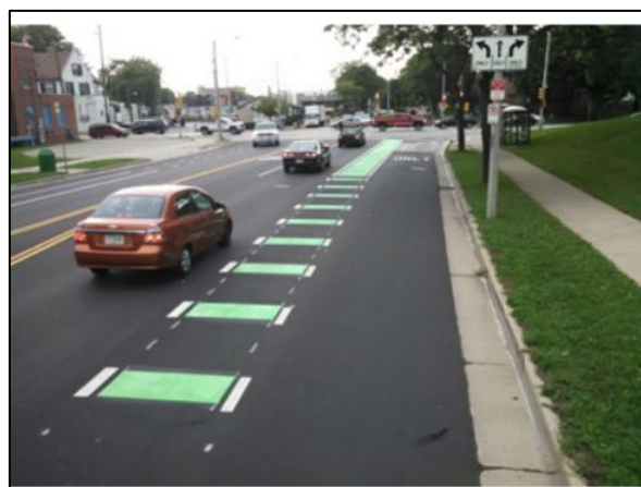
Figure 14: Example of Green Pavement Markings
