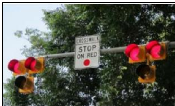
Figure 18: Example of a Pedestrian Hybrid Beacon Mounted on a Mast Arm
