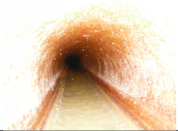
Inlet Pipe: P1
