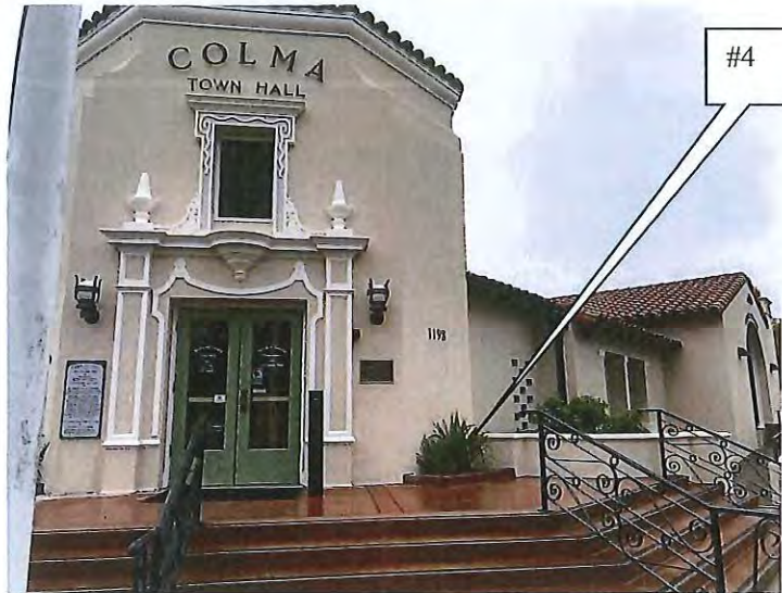
78. Typical planters along Town Hall Frontage.
