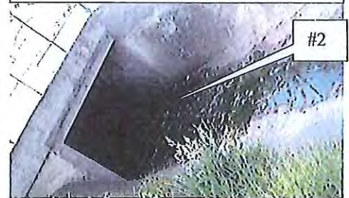
132. COLMA CREEK GOING UNDER SERRAMONTE BLVD.
