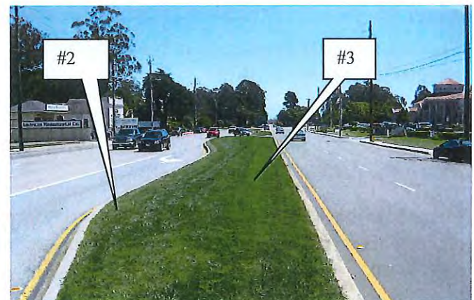
5. EL CAMINO REAL AT COLLINS AVE VIEWING SOUTH "THE Y" (VIEWING SOUTH)
