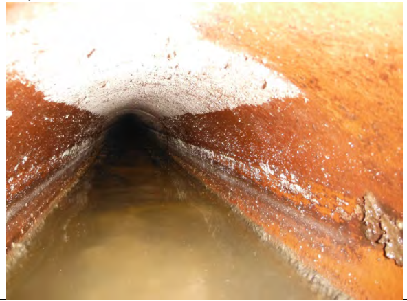
Inlet Pipe: P1
