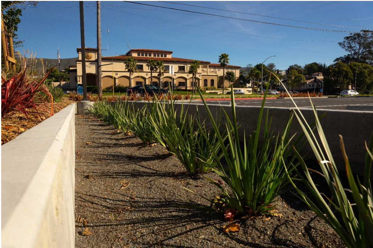
Bioretention area located at Town Hall.
