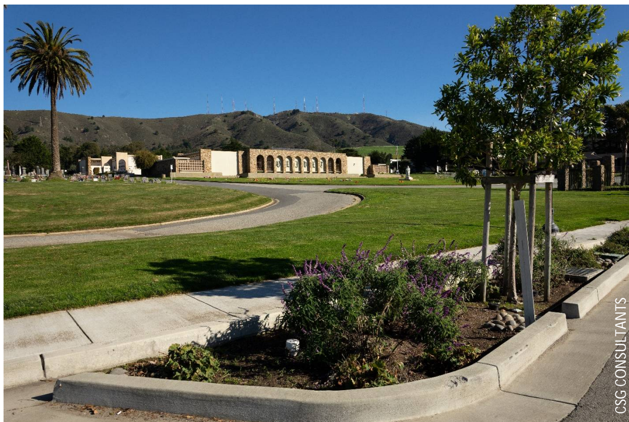
Bioretention curb extension located at Hillside Boulevard.
