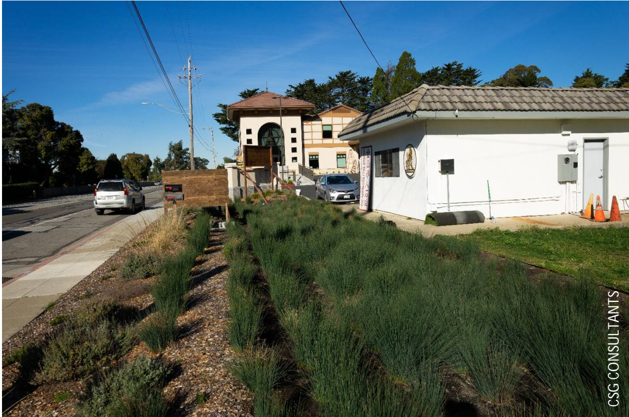
Bioretention area located at Golden Hills Memorial Park.
