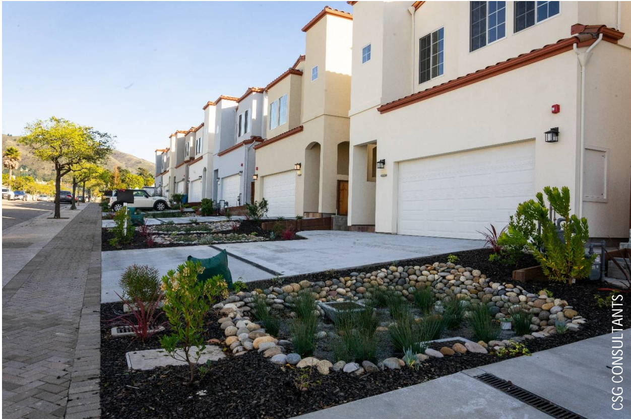
Bioretention areas located at B Street.
