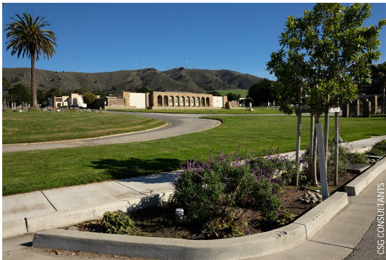
Bioretention curb extension located at Hillside Boulevard.
