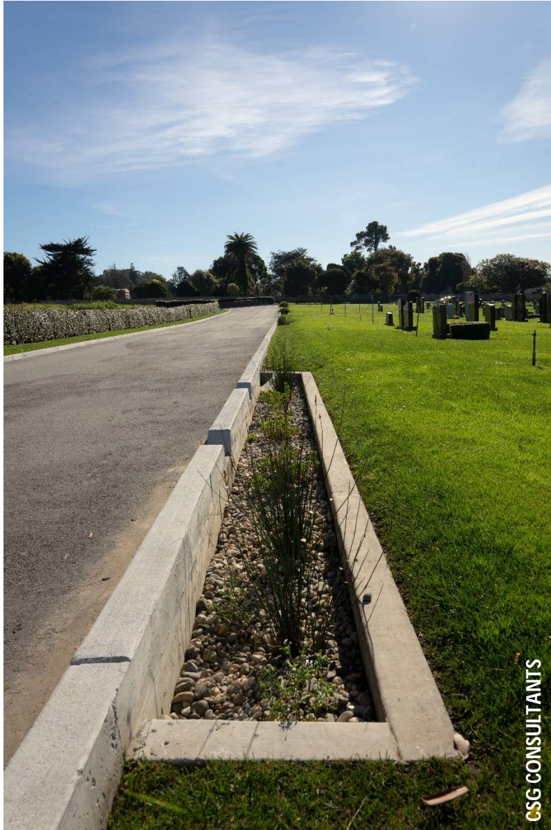
Bioretention Area located at Hills of Eternity.
