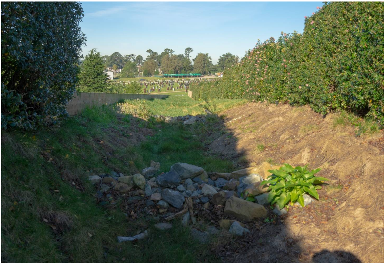
Bioretention area located at Cypress Lawn.
