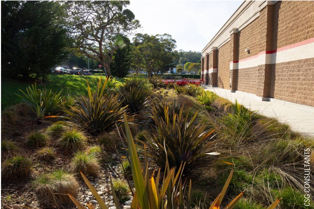
Bioretention area located at Target in Serramonte Shopping Center.
