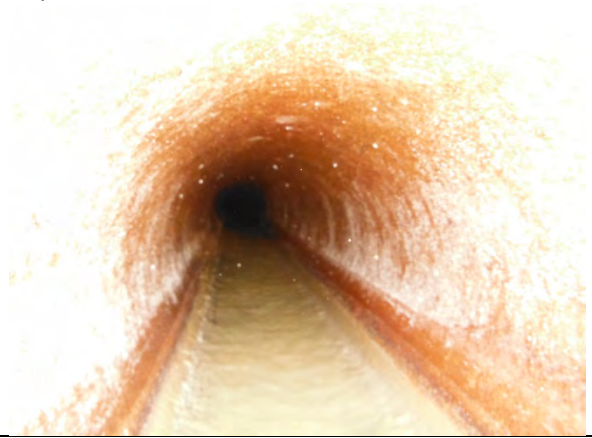
Inlet Pipe: P1
