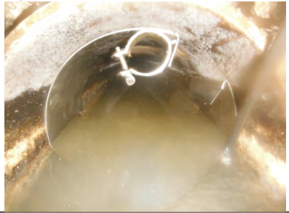
Inlet Pipe: P1
