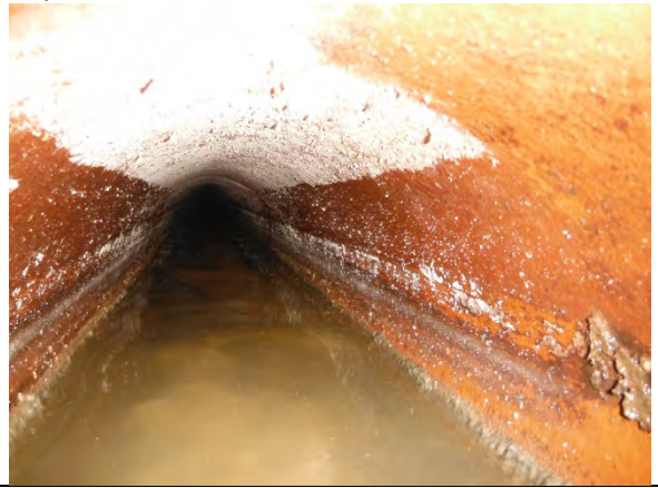
Inlet Pipe: P1
