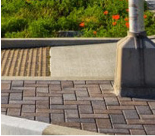
Existing Pavers, Hillside Blvd
