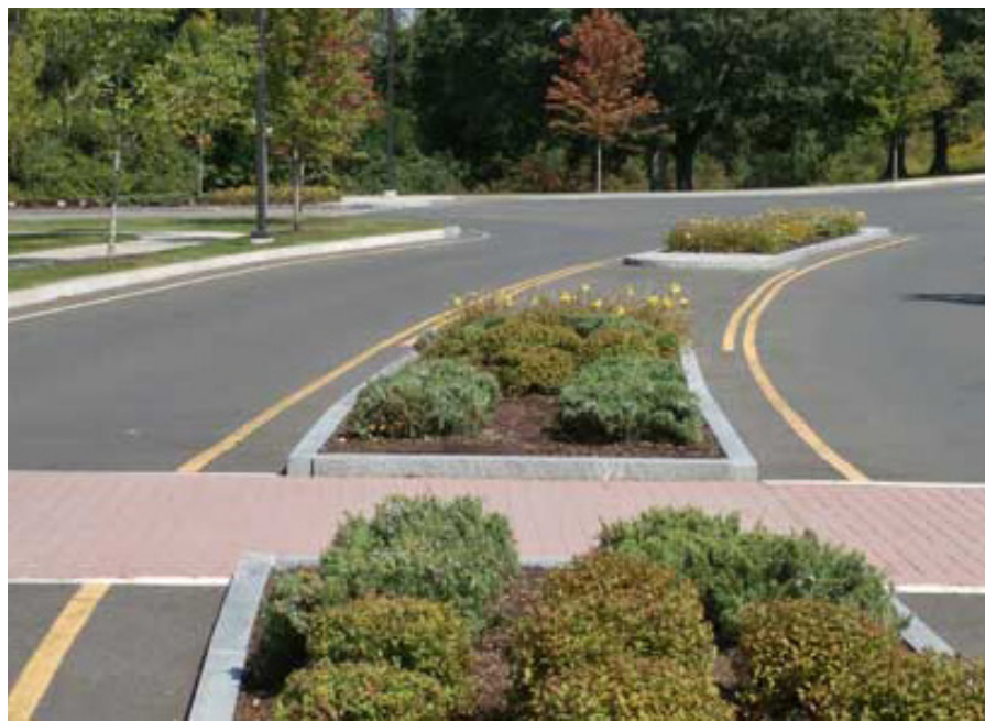
Pedestrian crossing refuge
