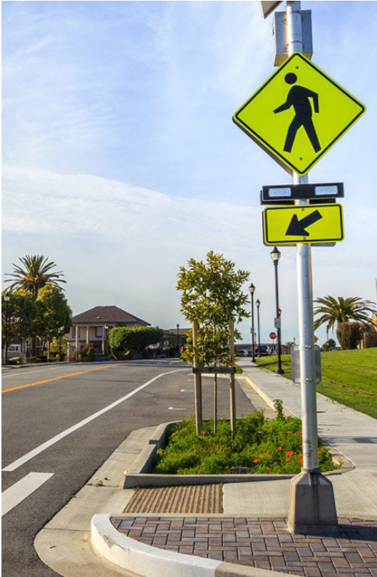
Existing Beacon and Detectable Warning Pavers Hillside Boulevard SOURCE: CSG Consultants
