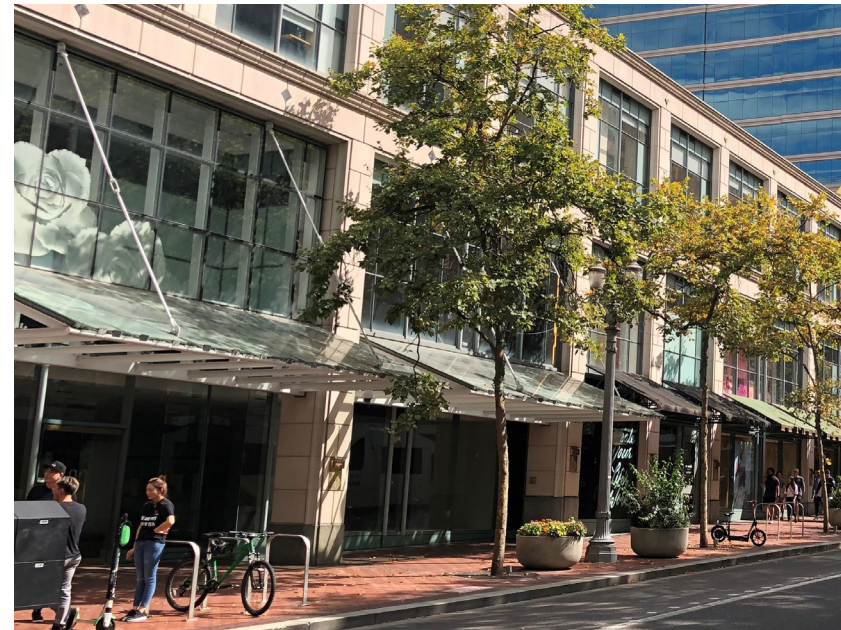
Example of Active Building Design
