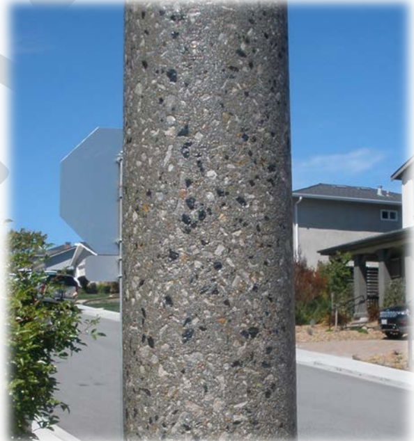
Round concrete light pole – San Bruno
